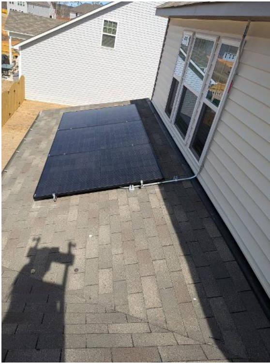
Roof Photos / Array 2 / Complete Array with all modules visible + Rail trimmed
