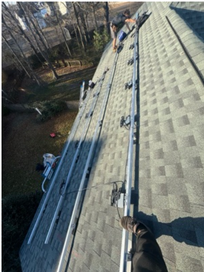
Detailed picture of installed MICRO inverters and wire management
