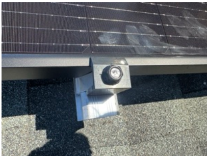
Detailed picture of END CLAMPS (with tape showing min 3/4" to edge of rail)
