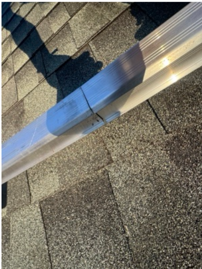
Detailed picture of rack splicing
