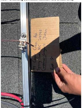
Roof / Grounding Connection between rails at each array
