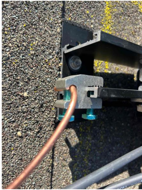
Rooftop Installation / Array Bonding/Grounding
