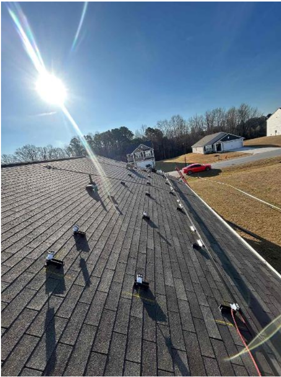
Rooftop Installation / Module Ready Photos
