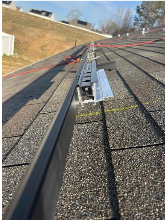
Rooftop Installation / Close Up of Skirt Splice + Skirt Roof Attachment Complete
