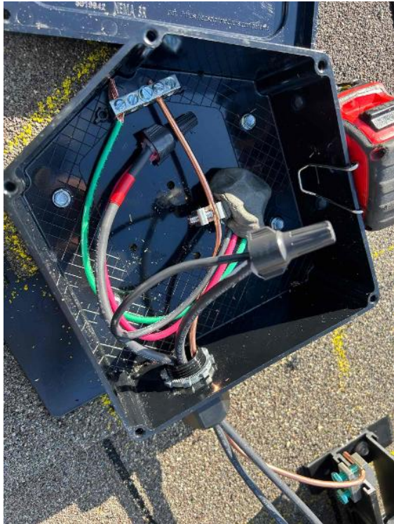
Rooftop Installation / Every J-Box Installed W/ Wiring Complete (All Components)
