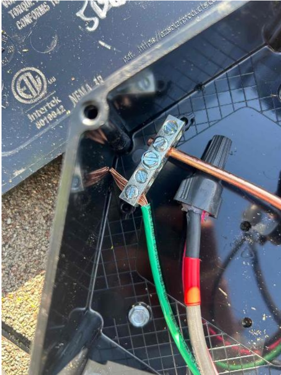
Rooftop Installation / Array Bonding/Grounding
