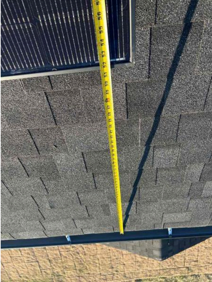
Inspection Photos: 183 Bering Cir, Angier, NC 27501 (Killgore)
