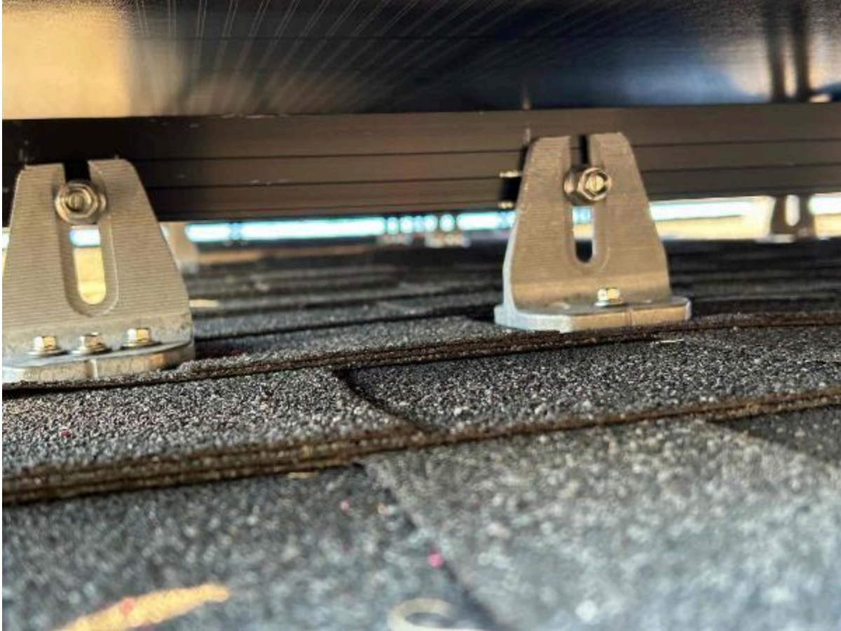
Inspection Photos: 183 Bering Cir, Angier, NC 27501 (Killgore)
