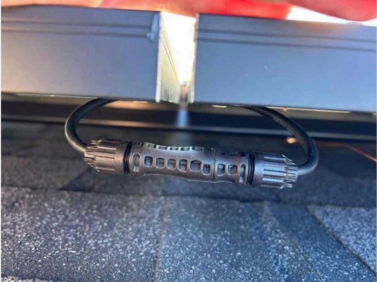
Inspection Photos: 183 Bering Cir, Angier, NC 27501 (Killgore)
