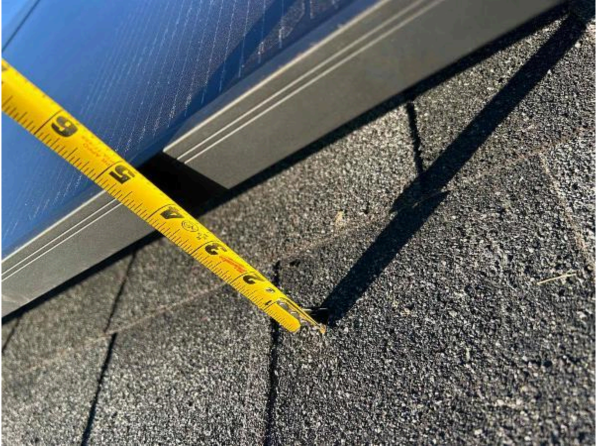
Inspection Photos: 183 Bering Cir, Angier, NC 27501 (Killgore)
