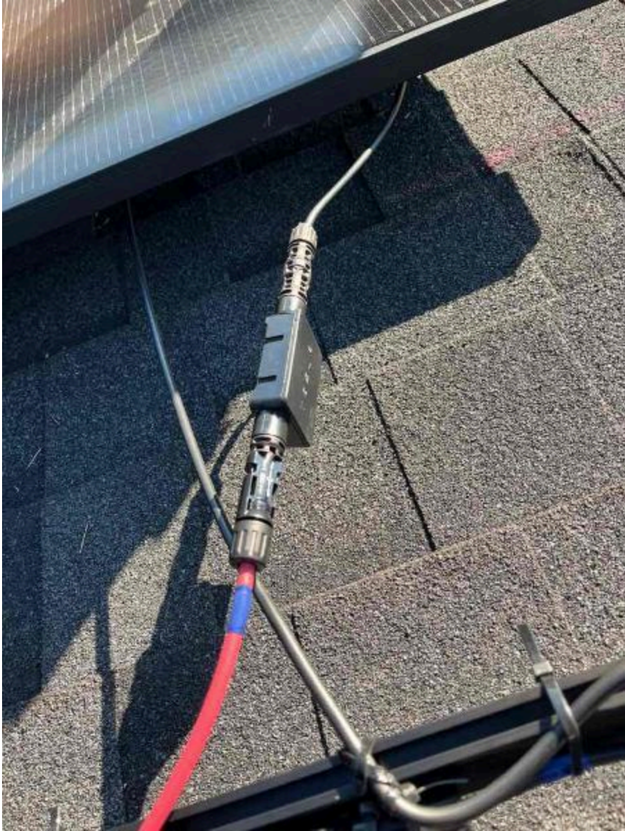
Inspection Photos: 183 Bering Cir, Angier, NC 27501 (Killgore)
