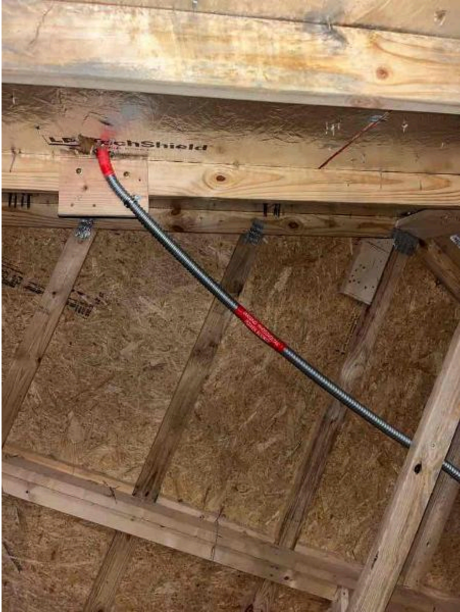
Inspection Photos: 183 Bering Cir, Angier, NC 27501 (Killgore)
