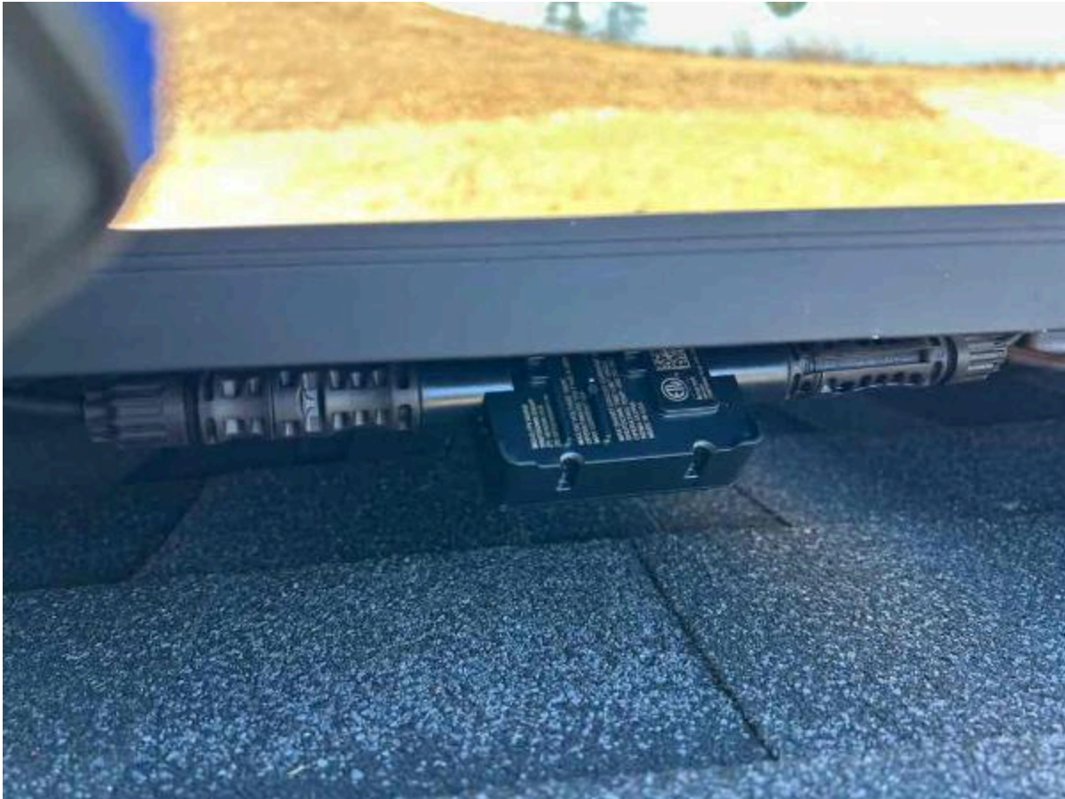
Inspection Photos: 183 Bering Cir, Angier, NC 27501 (Killgore)
