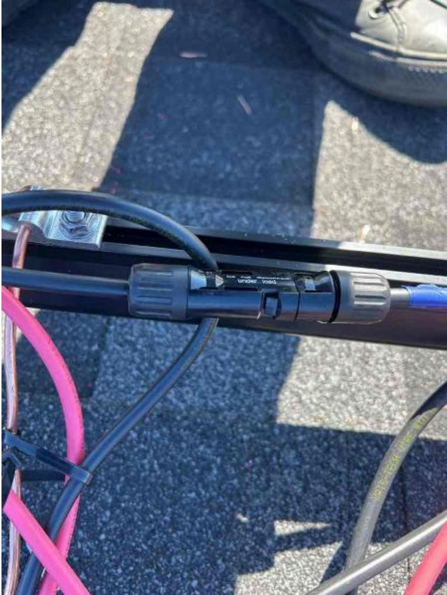
Inspection Photos: 183 Bering Cir, Angier, NC 27501 (Killgore)
