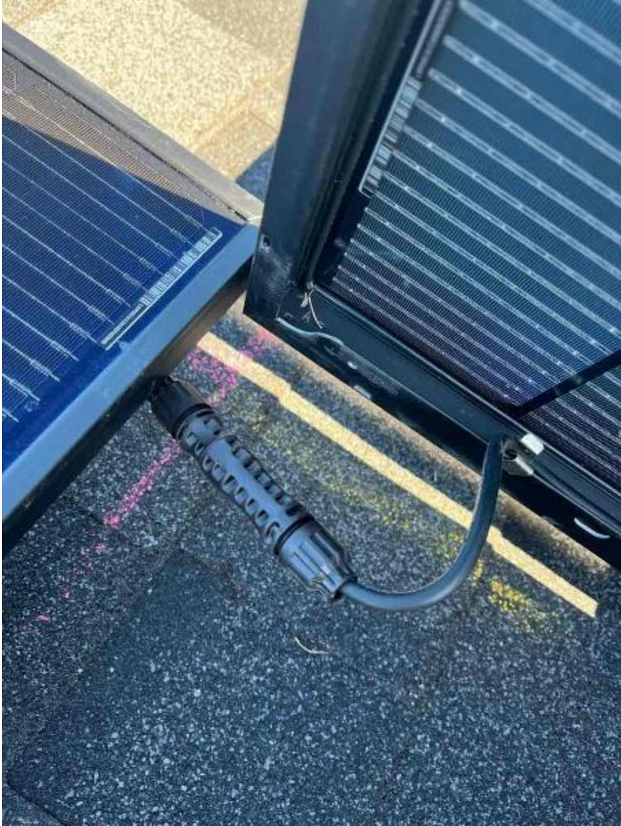
Inspection Photos: 183 Bering Cir, Angier, NC 27501 (Killgore)
