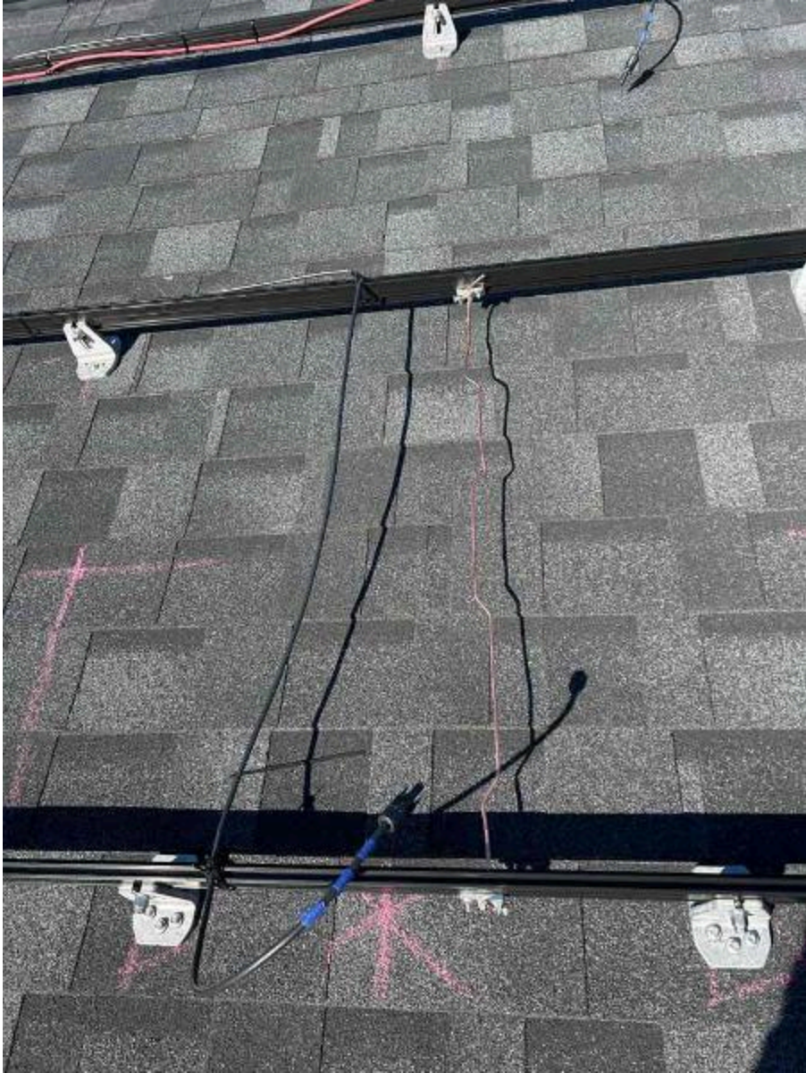
Inspection Photos: 183 Bering Cir, Angier, NC 27501 (Killgore)
