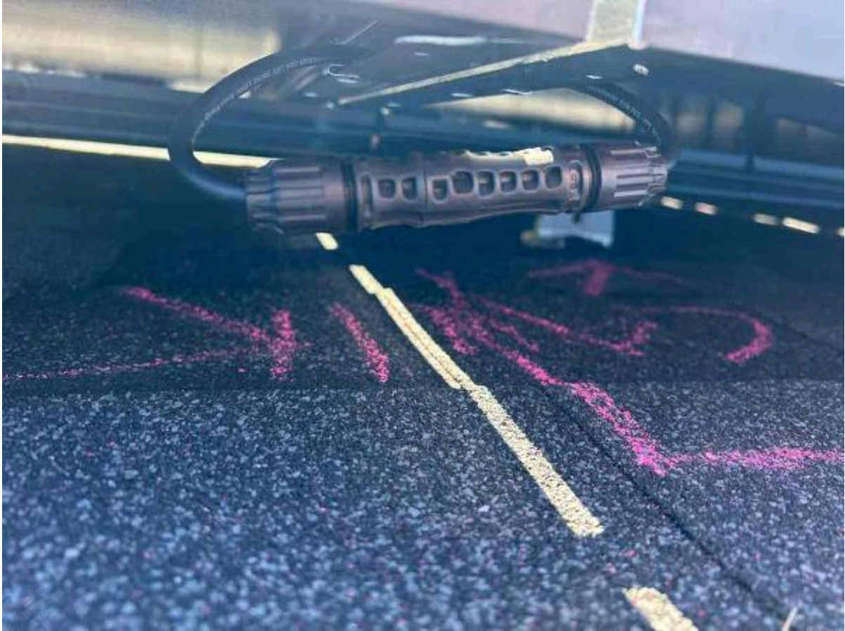
Inspection Photos: 183 Bering Cir, Angier, NC 27501 (Killgore)
