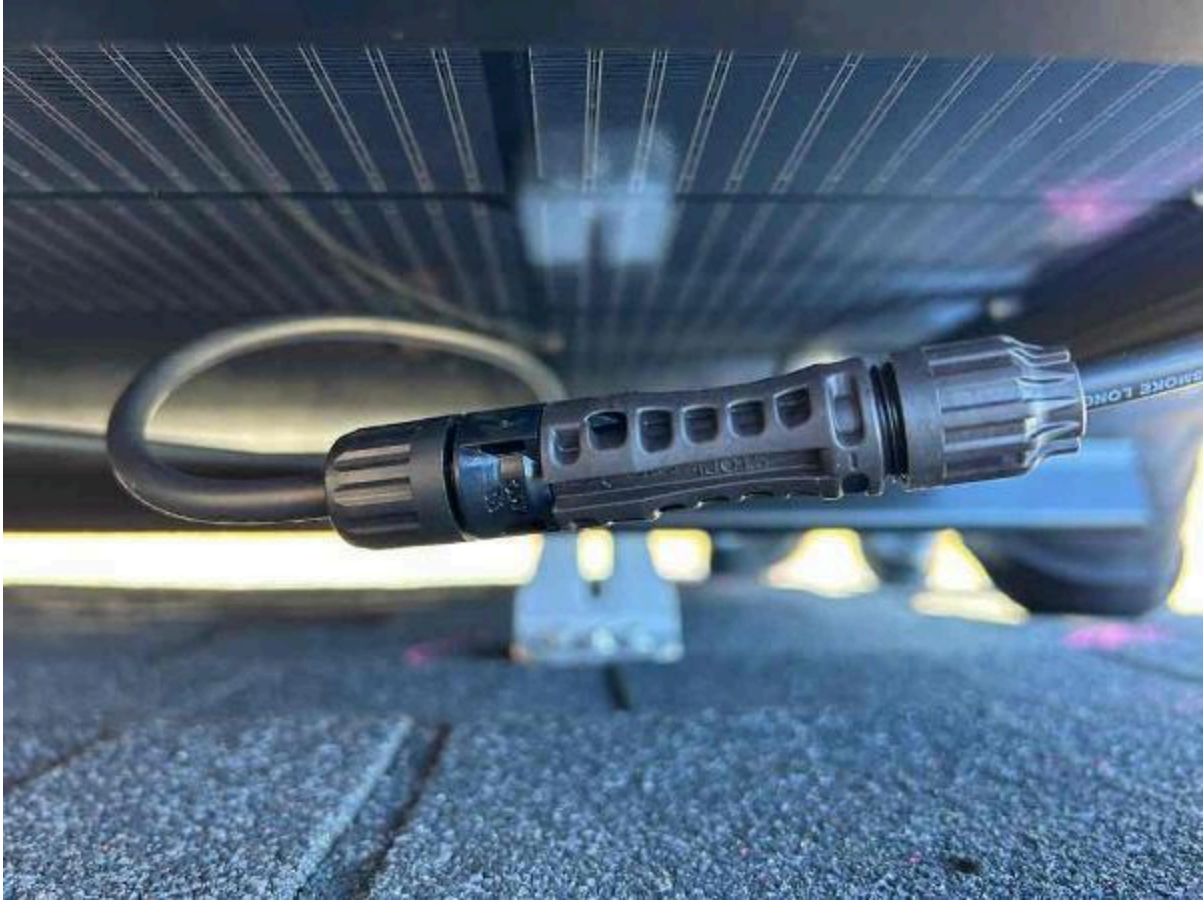
Inspection Photos: 183 Bering Cir, Angier, NC 27501 (Killgore)
