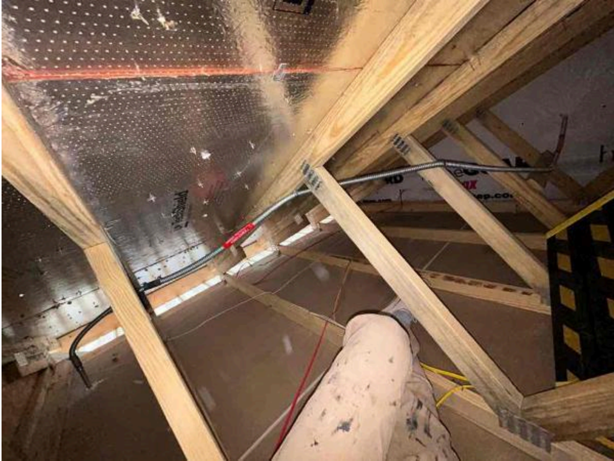
Inspection Photos: 183 Bering Cir, Angier, NC 27501 (Killgore)
