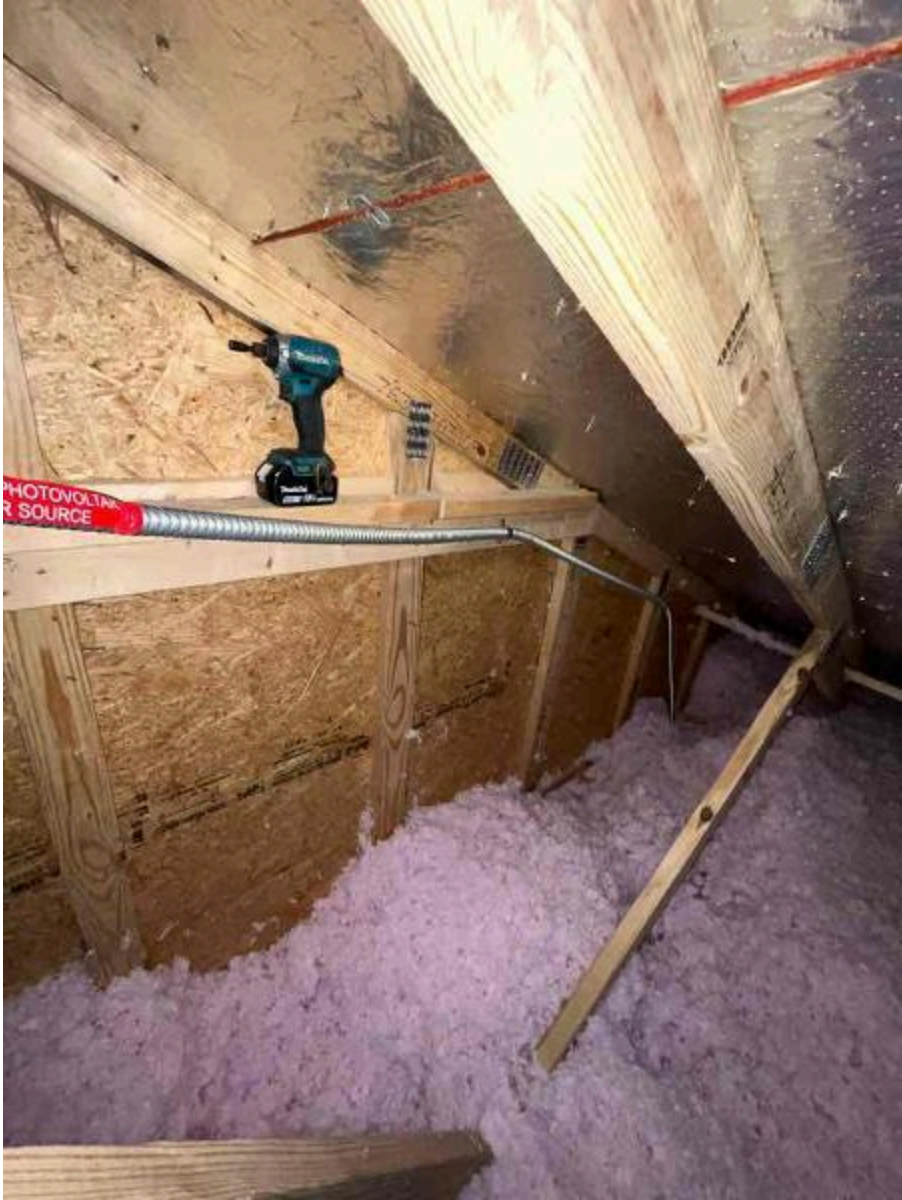
Inspection Photos: 183 Bering Cir, Angier, NC 27501 (Killgore)
