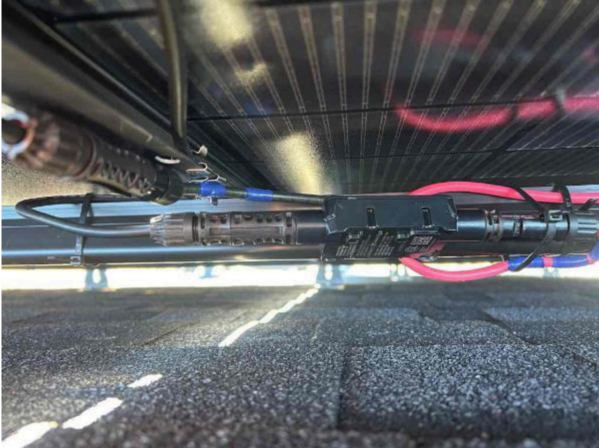
Inspection Photos: 183 Bering Cir, Angier, NC 27501 (Killgore)
