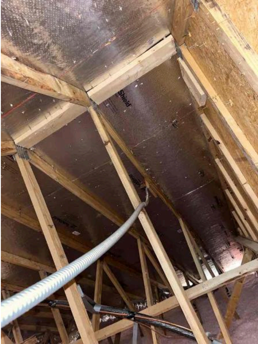
Inspection Photos: 183 Bering Cir, Angier, NC 27501 (Killgore)
