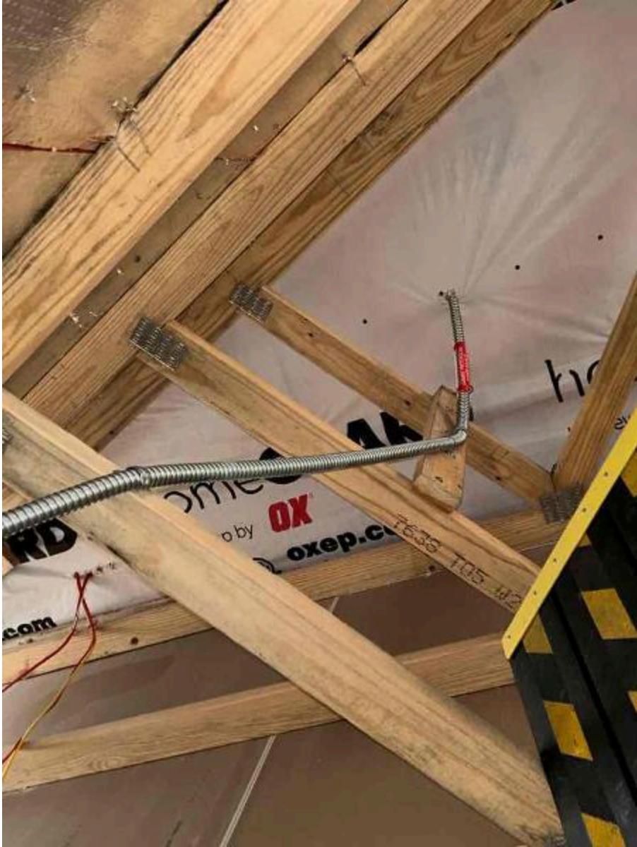
Inspection Photos: 183 Bering Cir, Angier, NC 27501 (Killgore)
