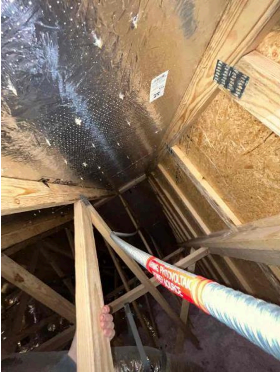
Inspection Photos: 183 Bering Cir, Angier, NC 27501 (Killgore)
