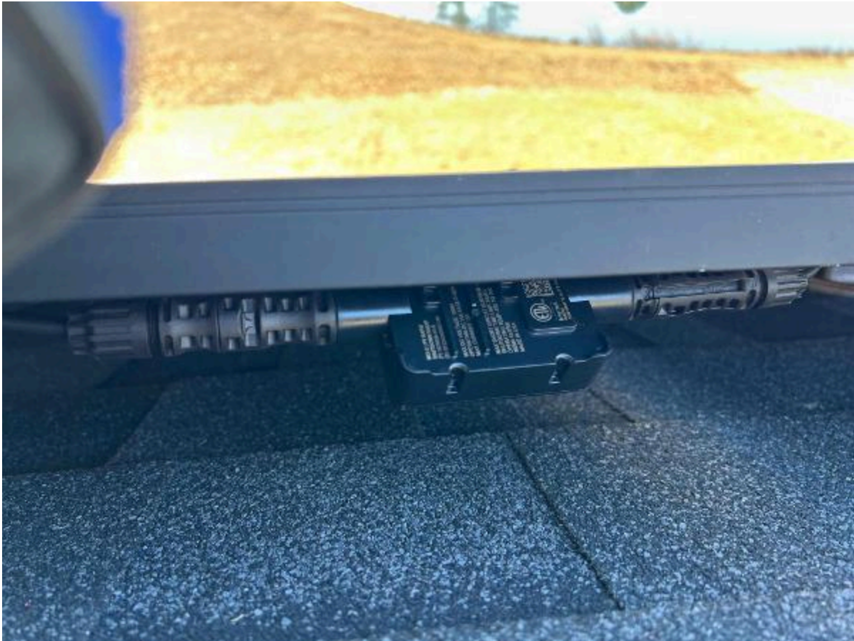
Inspection Photos: 183 Bering Cir, Angier, NC 27501 (Killgore)
