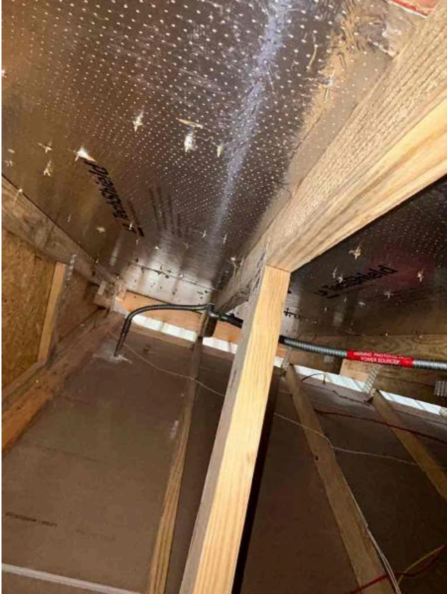
Inspection Photos: 183 Bering Cir, Angier, NC 27501 (Killgore)
