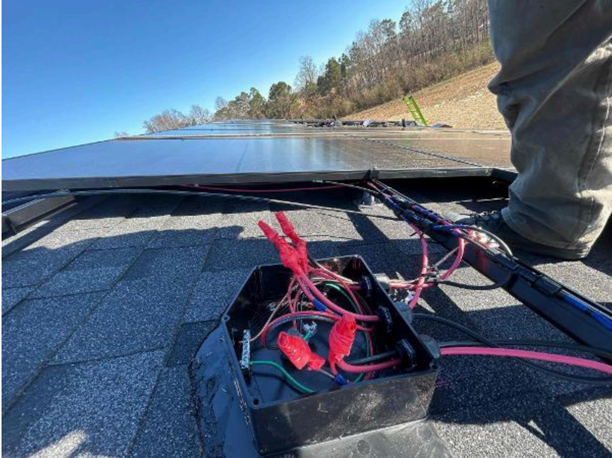
Inspection Photos: 183 Bering Cir, Angier, NC 27501 (Killgore)
