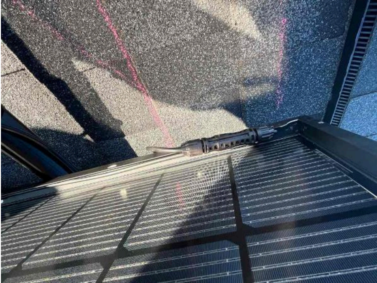
Inspection Photos: 183 Bering Cir, Angier, NC 27501 (Killgore)
