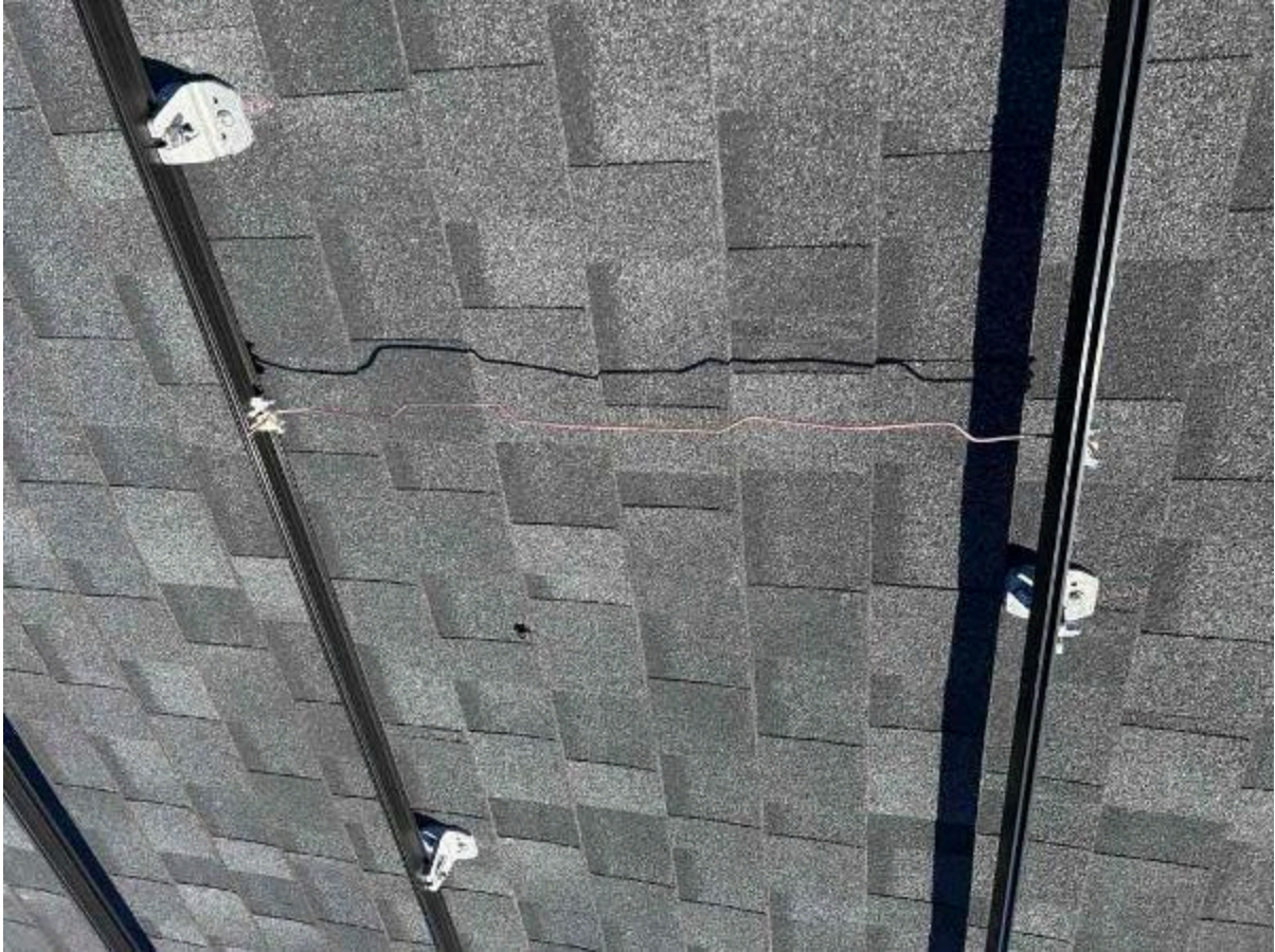
Inspection Photos: 183 Bering Cir, Angier, NC 27501 (Killgore)
