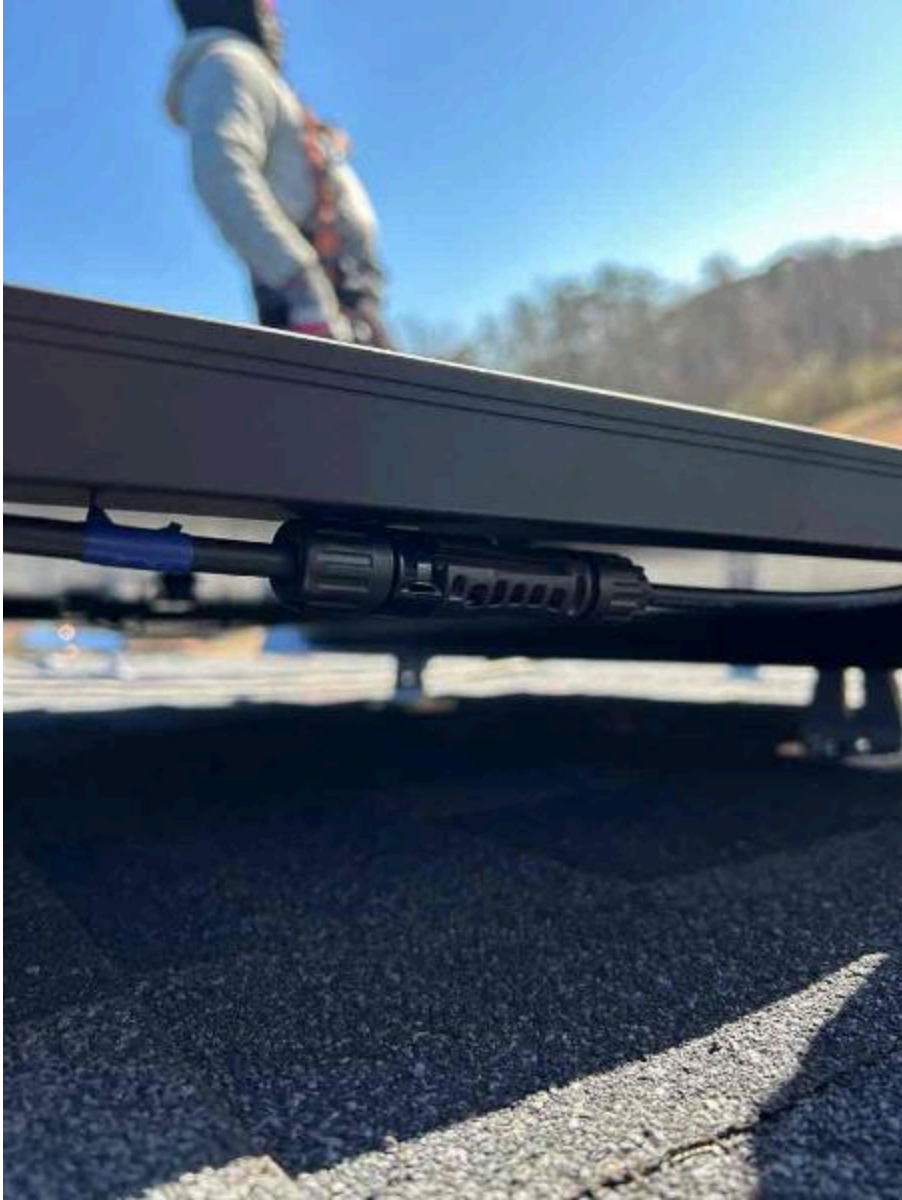
Inspection Photos: 183 Bering Cir, Angier, NC 27501 (Killgore)
