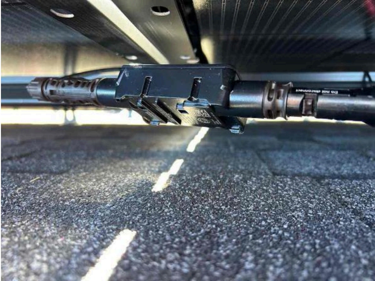
Inspection Photos: 183 Bering Cir, Angier, NC 27501 (Killgore)
