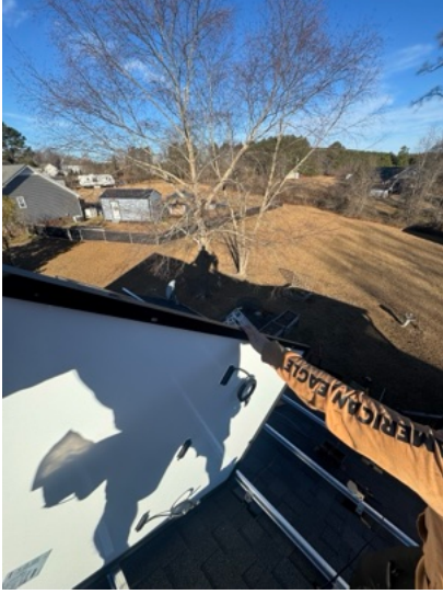
Detailed picture of Solar Deck/boxes (showing grounding / sealed penetration / all connections)
