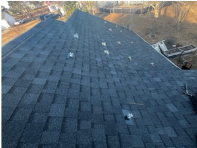
Detailed picture of installed FEET
