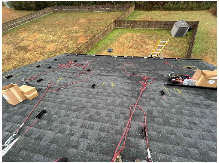
Rooftop Installation / Module Ready Photos
