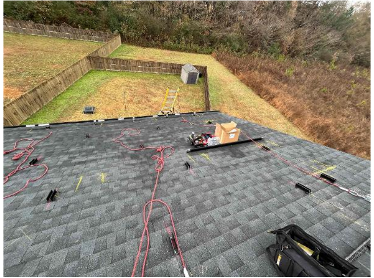
Rooftop Installation / Module Ready Photos
