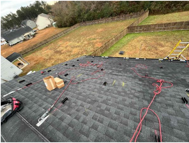
Rooftop Installation / Module Ready Photos
