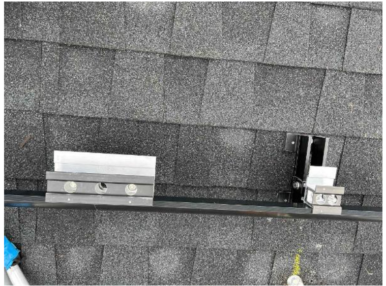
Rooftop Installation / Close Up of Railless Coupling Installed
