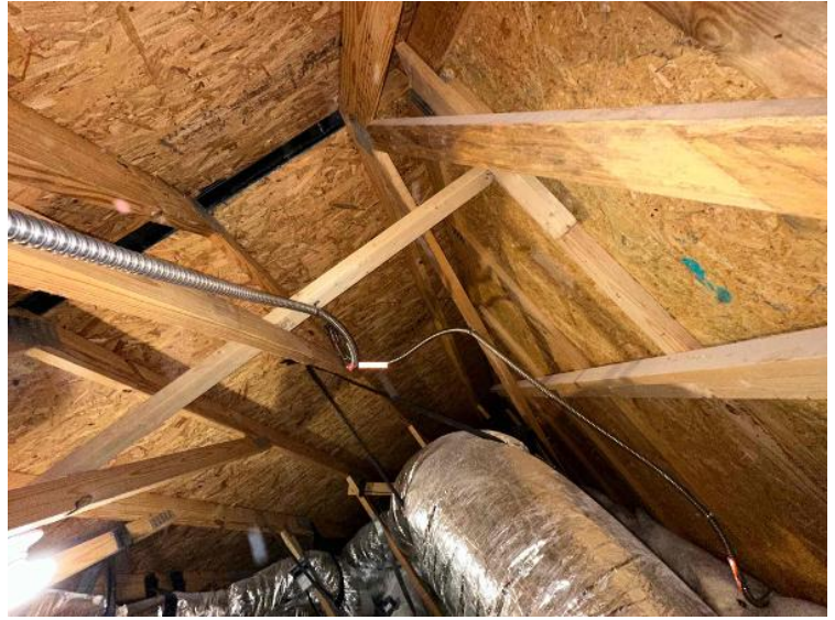
Rooftop Installation / Entire Attic Run
