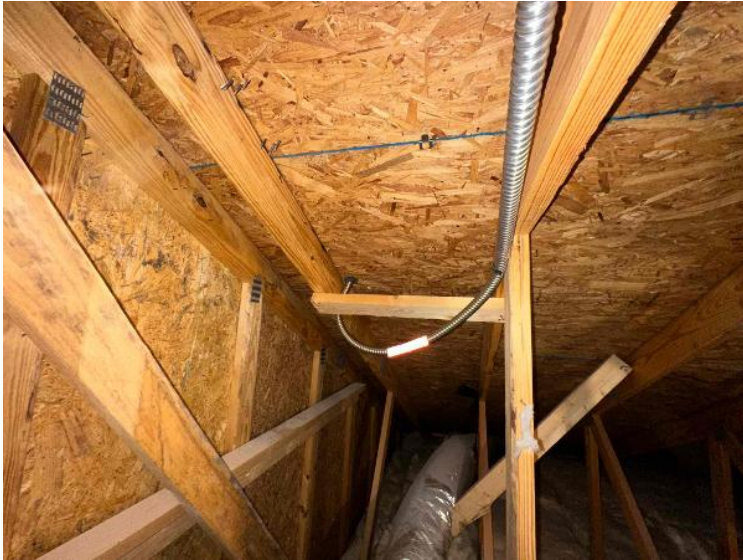
Rooftop Installation / Entire Attic Run
