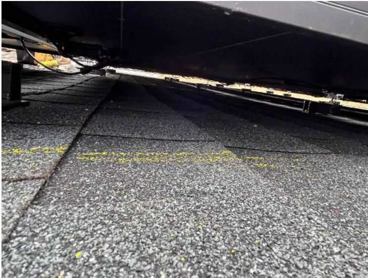
Rooftop Installation / Wire management Under the Array (1 photo per row of modules per array)
