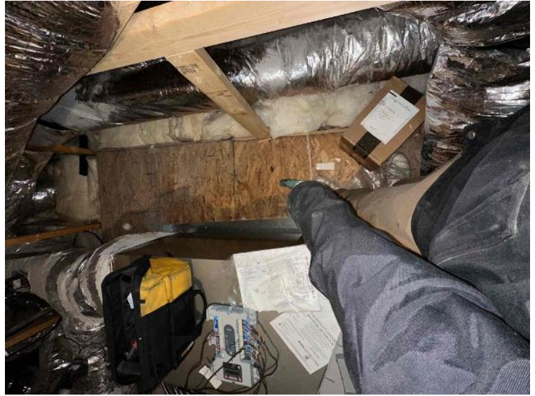
Rooftop Installation / Entire Attic Run
