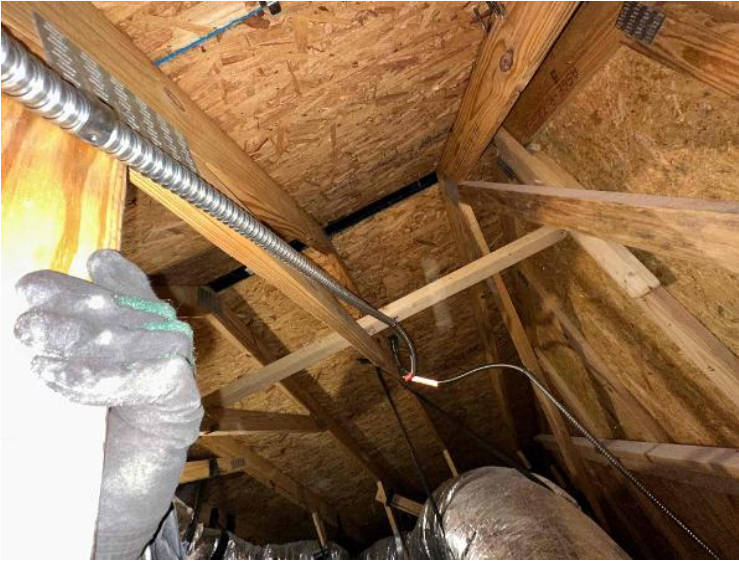
Rooftop Installation / Entire Attic Run
