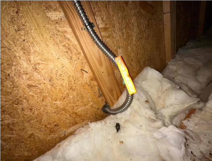
Rooftop Installation / Entire Attic Run
