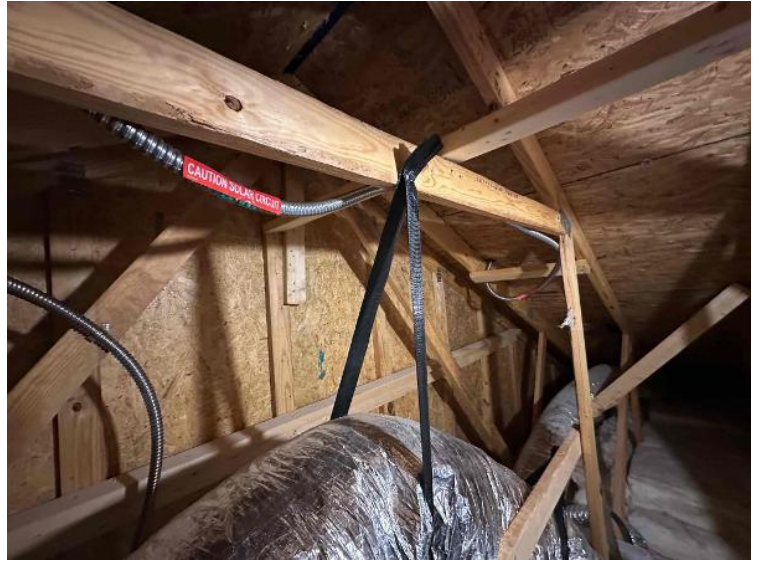
Rooftop Installation / Entire Attic Run
