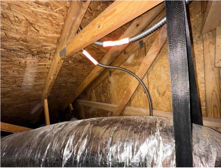
Rooftop Installation / Entire Attic Run
