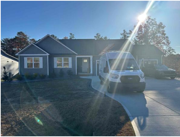
Job Check In / Picture of Front of the House with Address Visible
