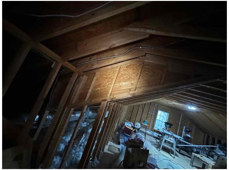
Rooftop Installation / Entire Attic Run
