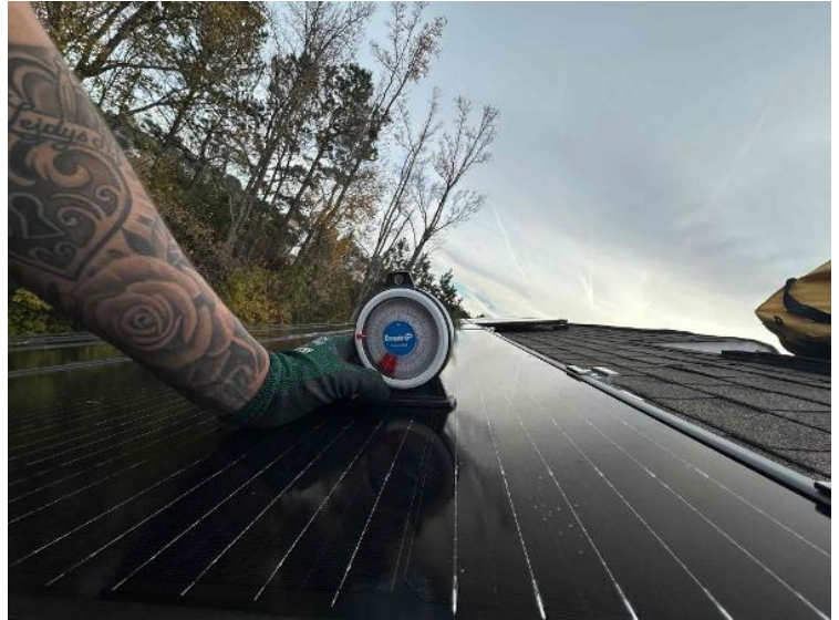
Project Completion Photos / Photo of array 1
