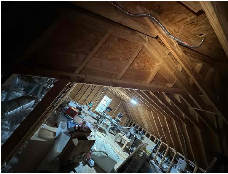
Rooftop Installation / Entire Attic Run
