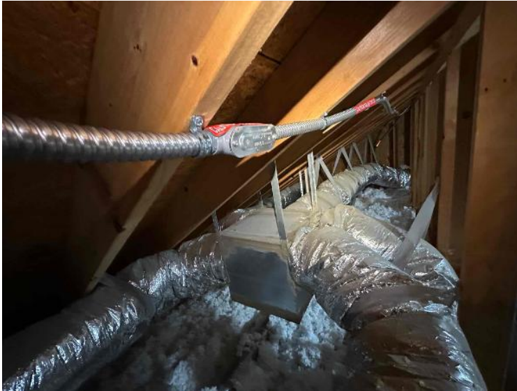
Rooftop Installation / Entire Attic Run
