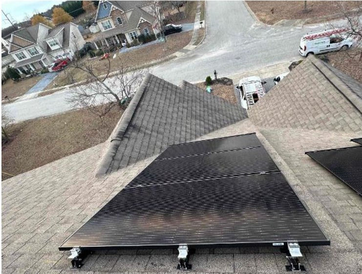
Project Completion Photos / Photo of array 3
