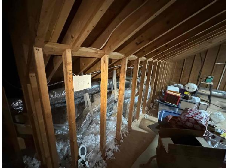
Rooftop Installation / Entire Attic Run
