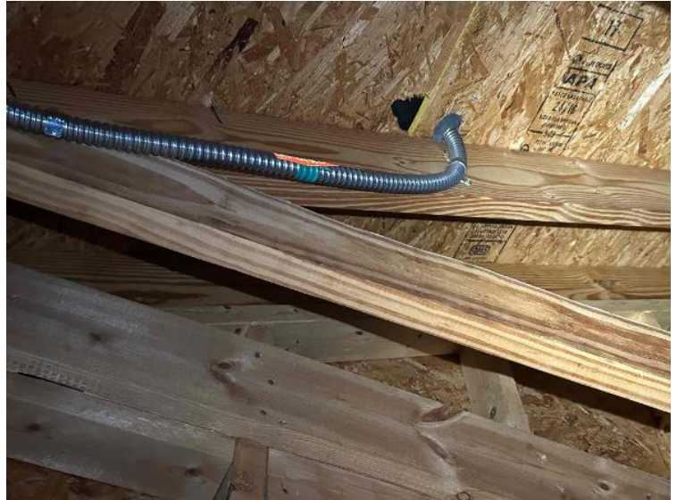
Rooftop Installation / Entire Attic Run
