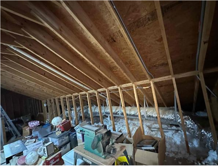
Rooftop Installation / Entire Attic Run
