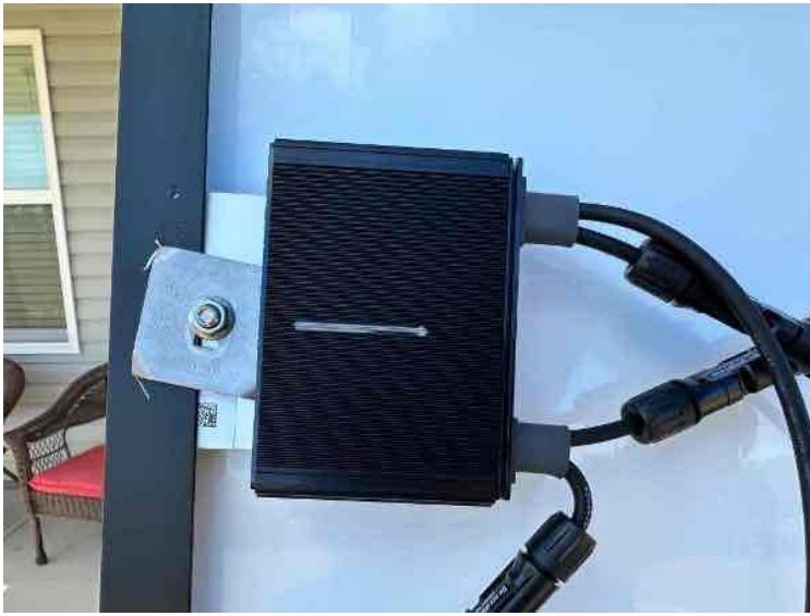
Rooftop Installation / 2 Optimizer's/ Micro Inverter's/ Tesla MCI's Installed
