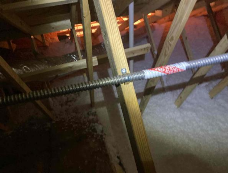
Rooftop Installation / Entire Attic Run
