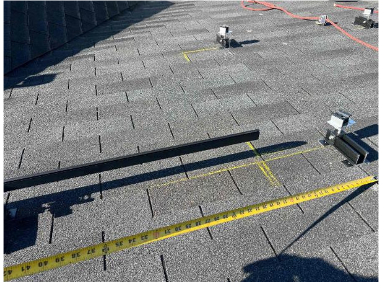
Rooftop Installation / Module Ready Photos
