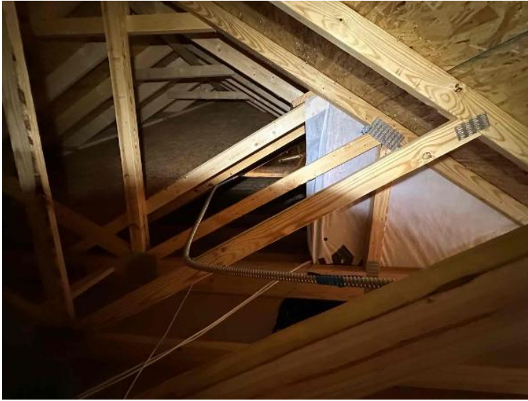
Rooftop Installation / Entire Attic Run
