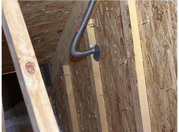
Rooftop Installation / Entire Attic Run
