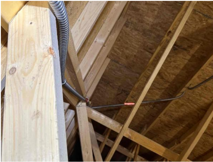
Rooftop Installation / Entire Attic Run
