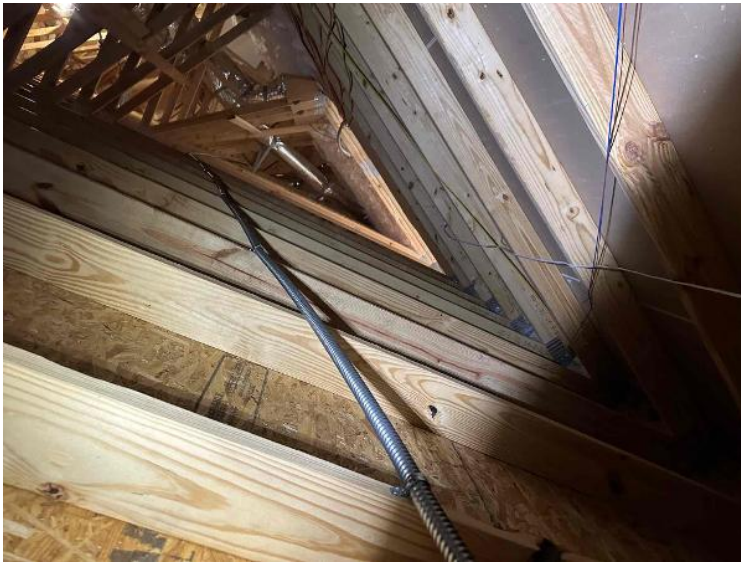
Rooftop Installation / Entire Attic Run
