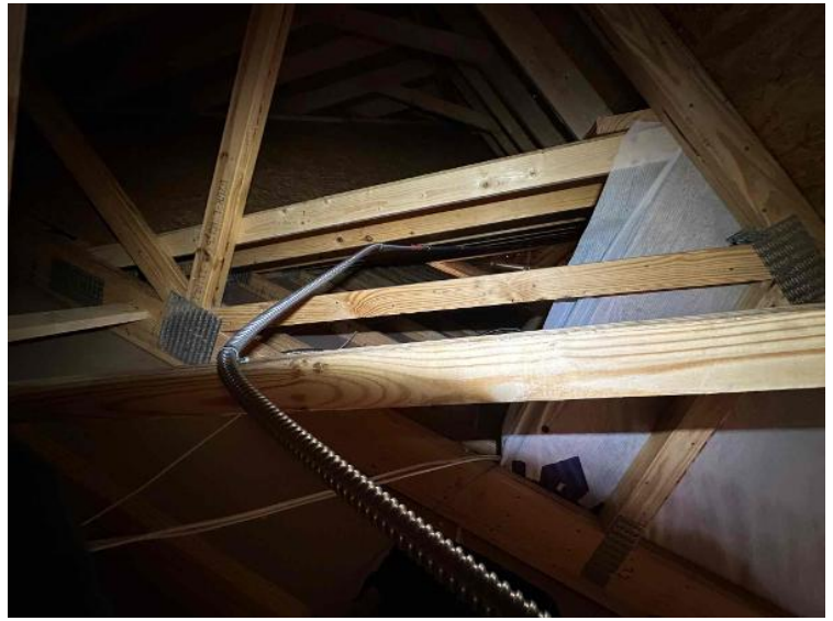
Rooftop Installation / Entire Attic Run
