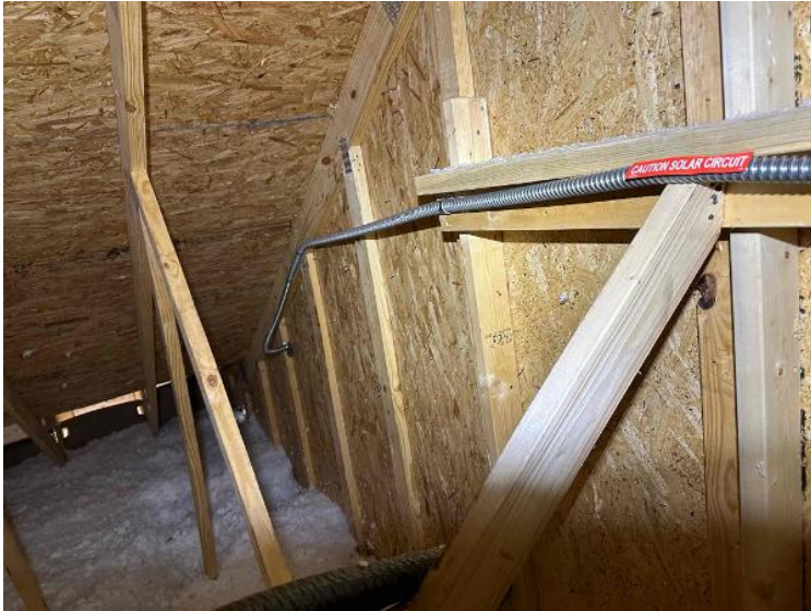
Rooftop Installation / Entire Attic Run
