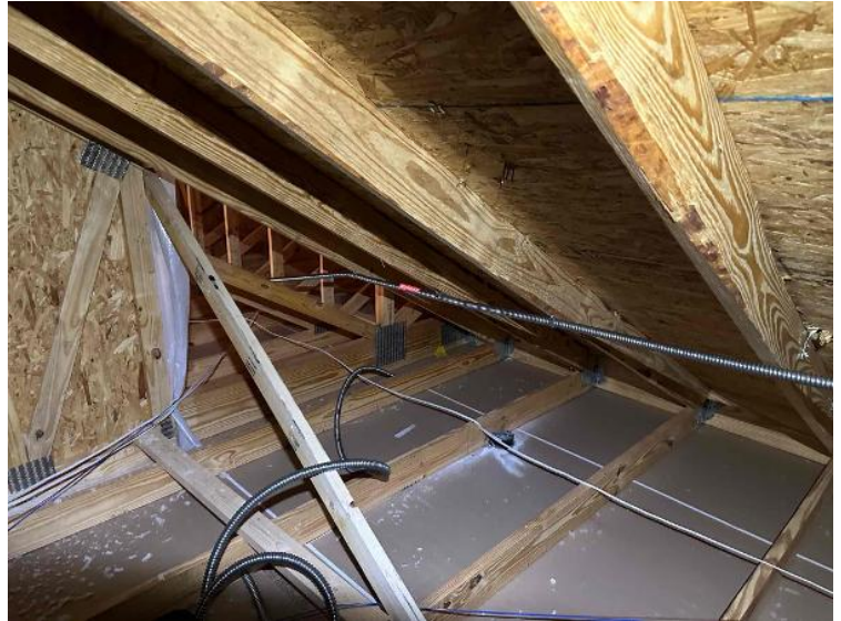
Rooftop Installation / Entire Attic Run
