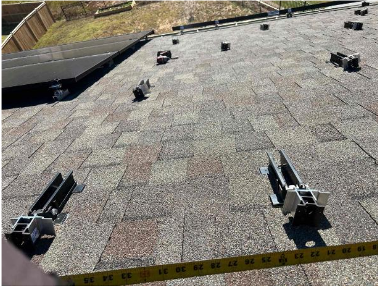
Rooftop Installation / Module Ready Photos
