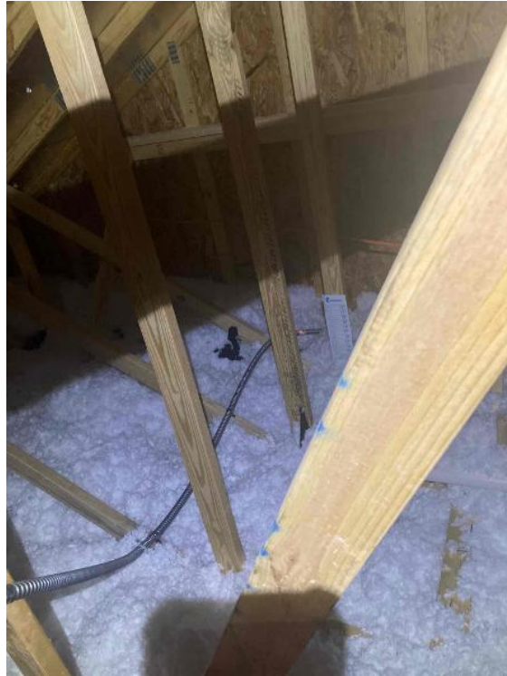
Rooftop Installation / Entire Attic Run
