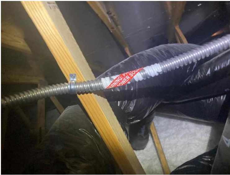
Rooftop Installation / Entire Attic Run
