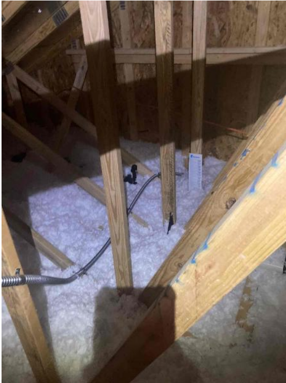
Rooftop Installation / Entire Attic Run
