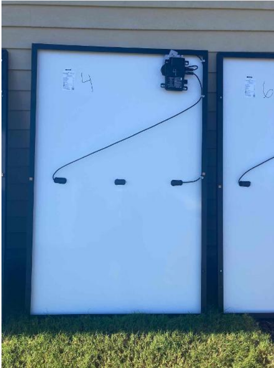
Rooftop Installation / 2 Optimizer's/ Micro Inverter's/ Tesla MCI's Installed
