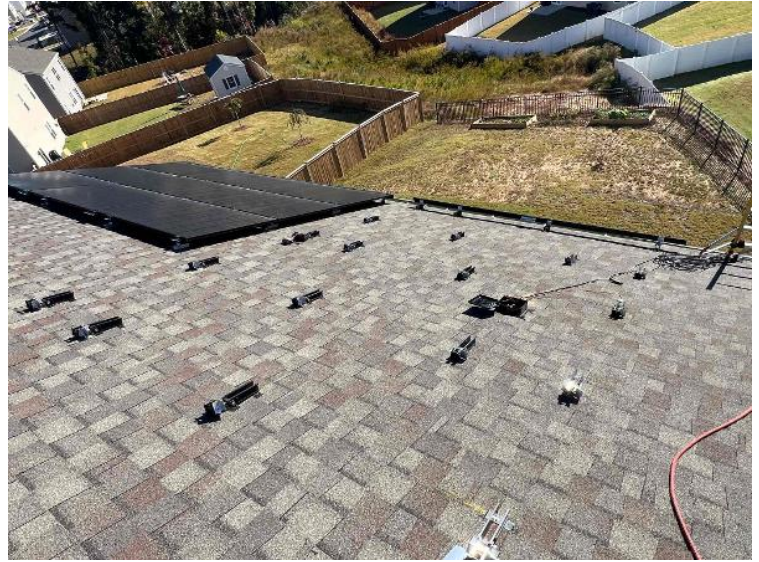
Rooftop Installation / Module Ready Photos
