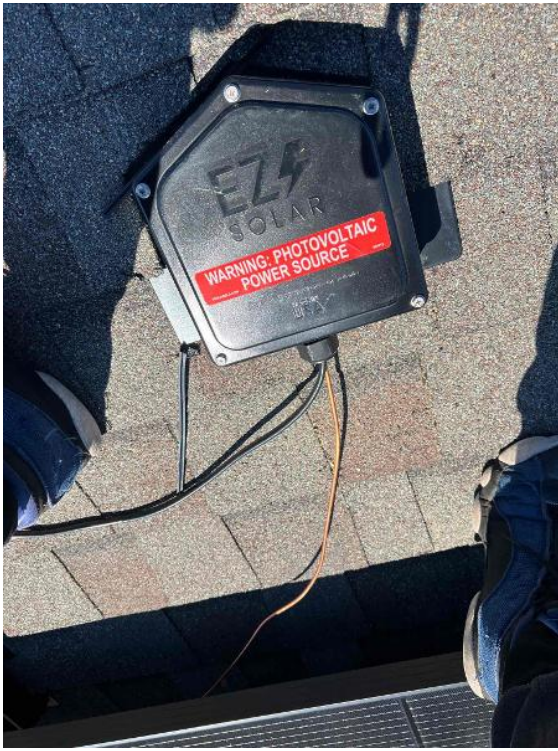
Rooftop Installation / J-Box Completed W/ Lid Installed
