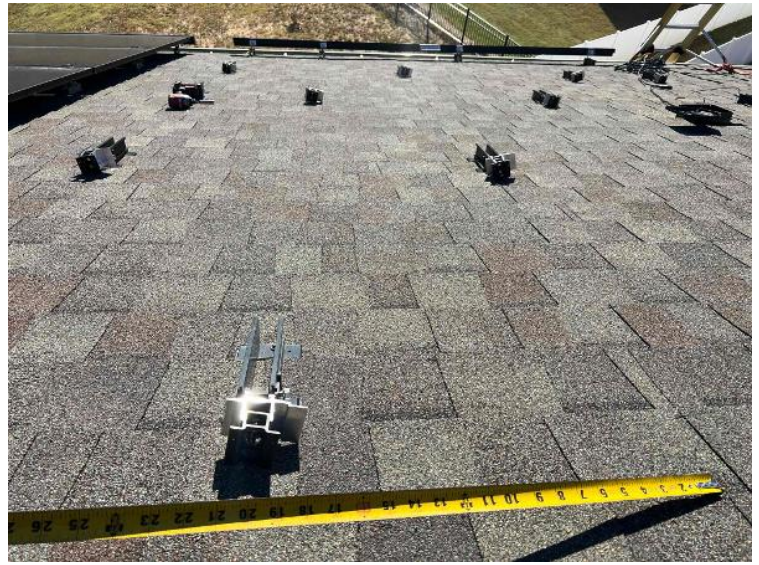
Rooftop Installation / Module Ready Photos
