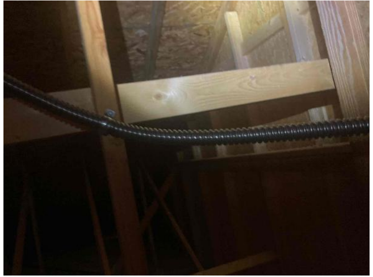
Rooftop Installation / Entire Attic Run
