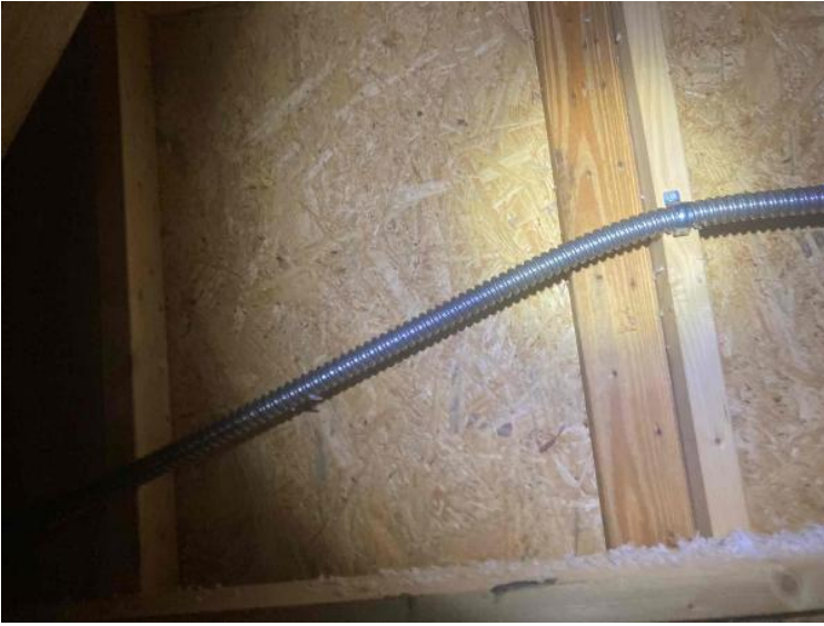
Rooftop Installation / Entire Attic Run
