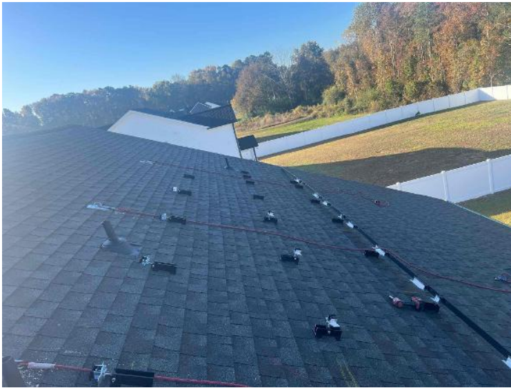
Rooftop Installation / Module Ready Photos
