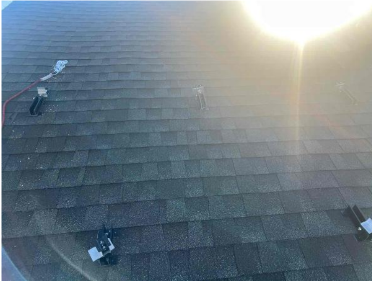
Rooftop Installation / Module Ready Photos
