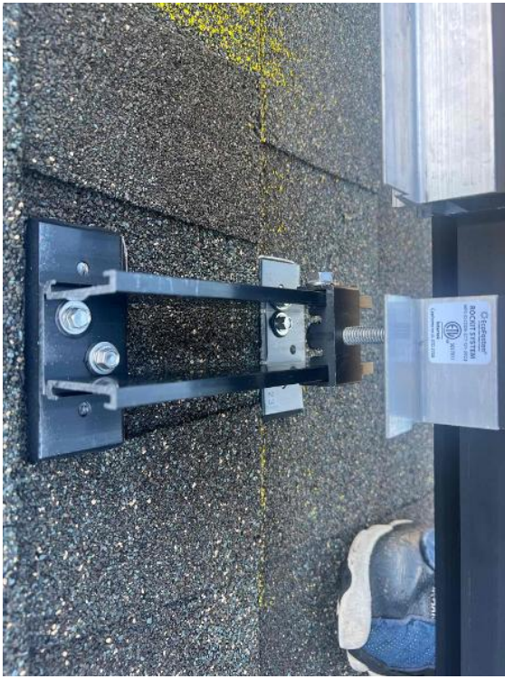
Rooftop Installation / Completed Roof Attachment
