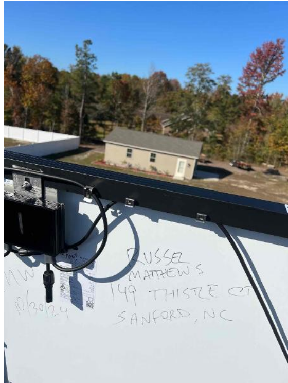
Rooftop Installation / Module Ready Photos
