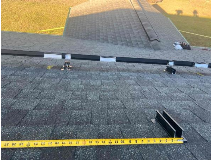
Rooftop Installation / Module Ready Photos
