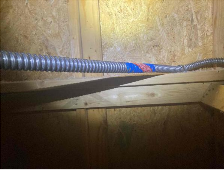
Rooftop Installation / Entire Attic Run
