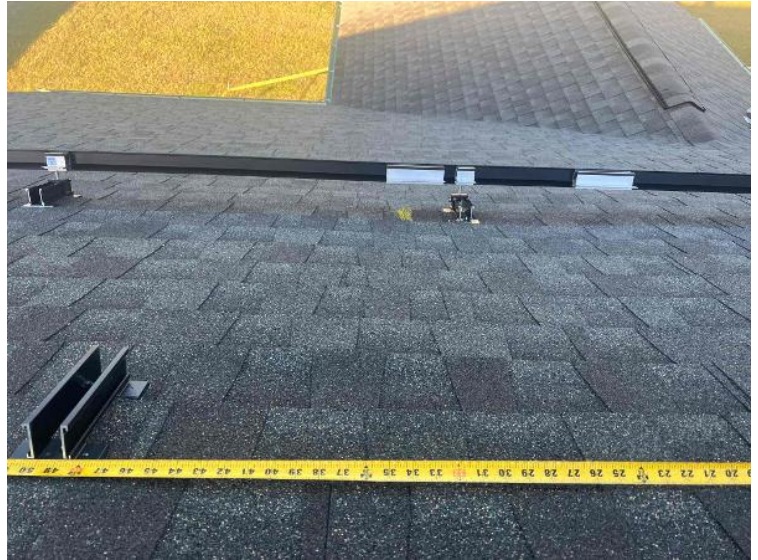
Rooftop Installation / Module Ready Photos
