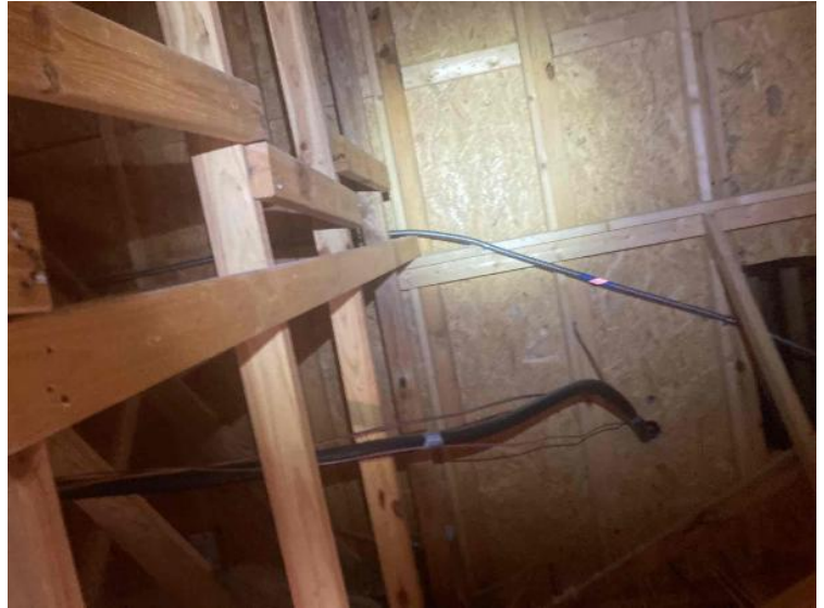
Rooftop Installation / Entire Attic Run
