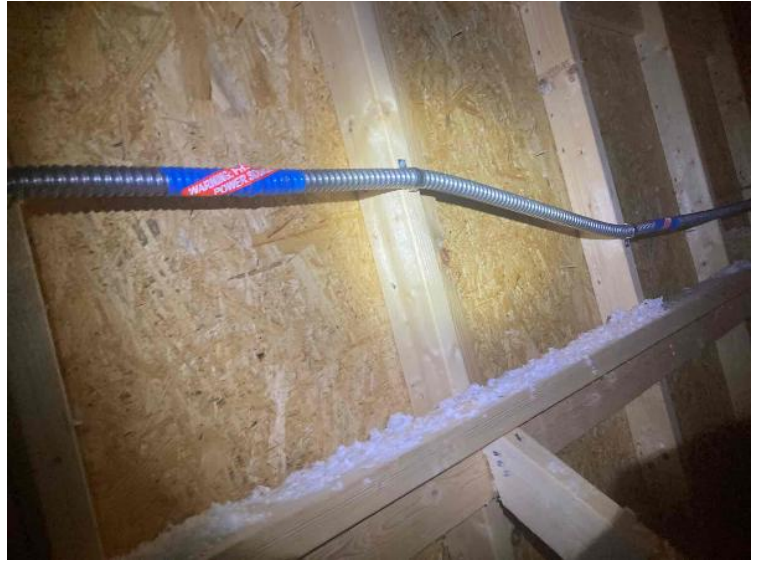
Rooftop Installation / Entire Attic Run
