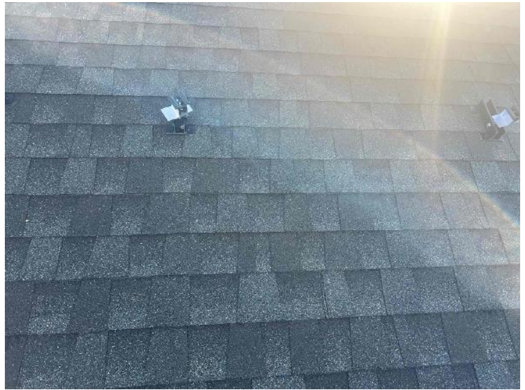
Rooftop Installation / Module Ready Photos
