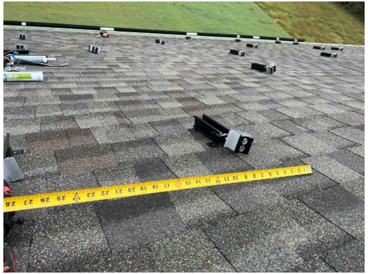
Rooftop Installation / Module Ready Photos
