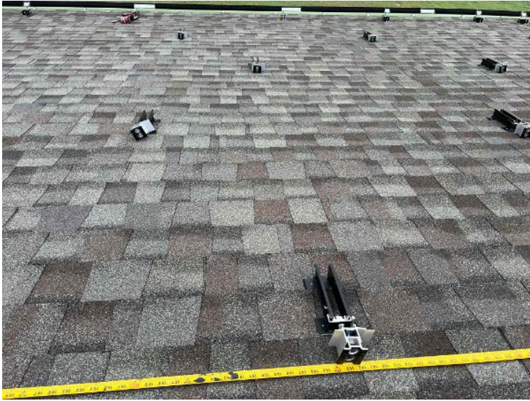
Rooftop Installation / Module Ready Photos
