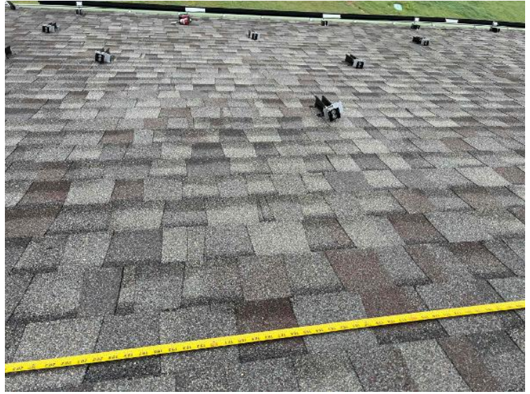
Rooftop Installation / Module Ready Photos
