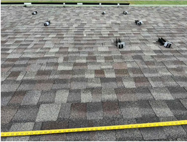
Rooftop Installation / Module Ready Photos
