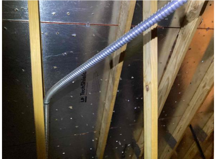
Rooftop Installation / Entire Attic Run
