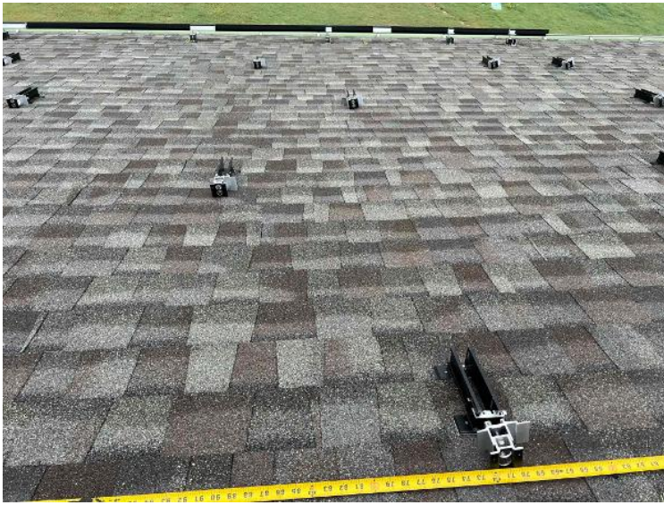
Rooftop Installation / Module Ready Photos
