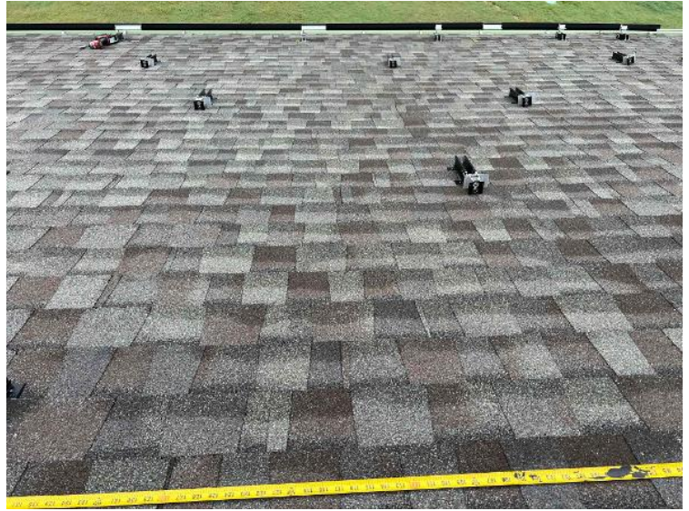
Rooftop Installation / Module Ready Photos
