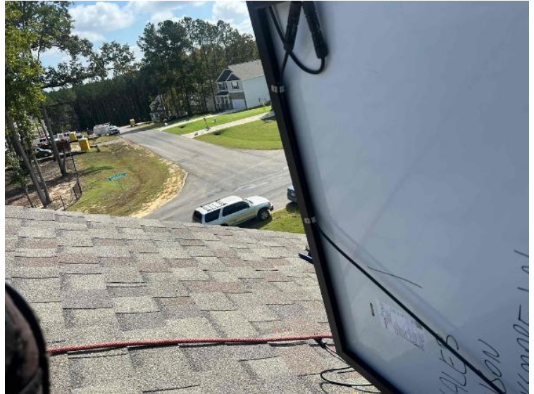
Rooftop Installation / Module Ready Photos
