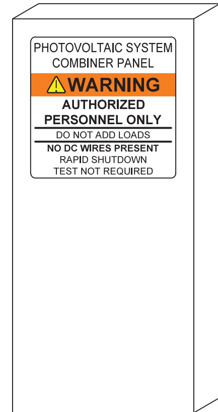
PV COMBINER BOX
