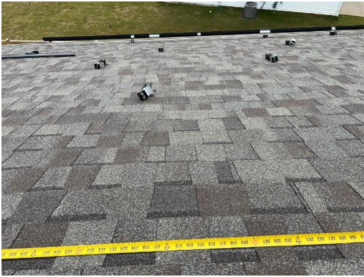
Rooftop Installation / Module Ready Photos
