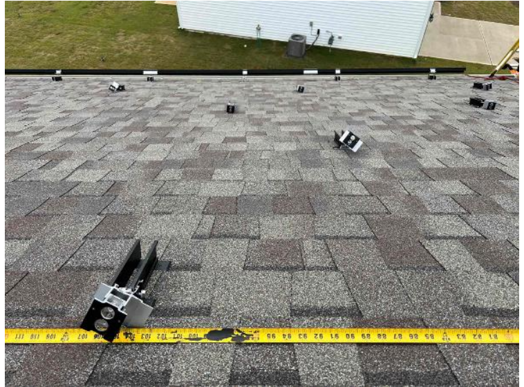
Rooftop Installation / Module Ready Photos
