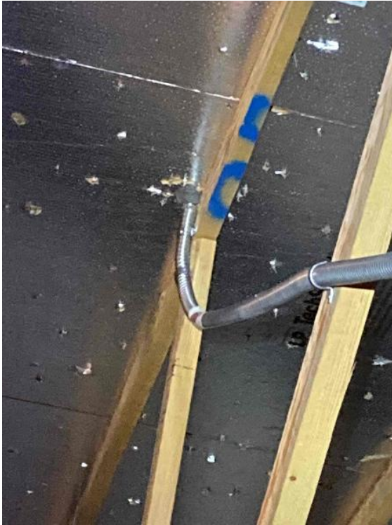
Rooftop Installation / Entire Attic Run
