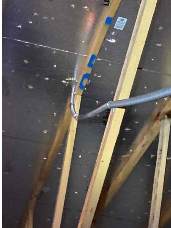
Rooftop Installation / Entire Attic Run
