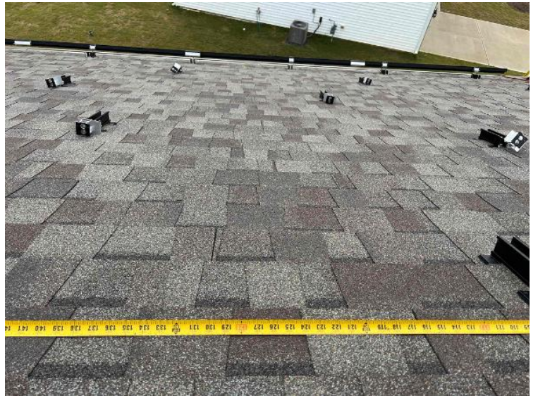
Rooftop Installation / Module Ready Photos
