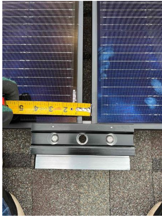
Rooftop Installation / Close Up of Railless Coupling Installed
