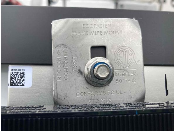
Rooftop Installation / Optimizer/ Micro Inverter Installed
