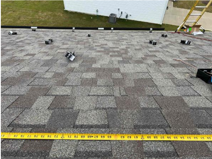
Rooftop Installation / Module Ready Photos
