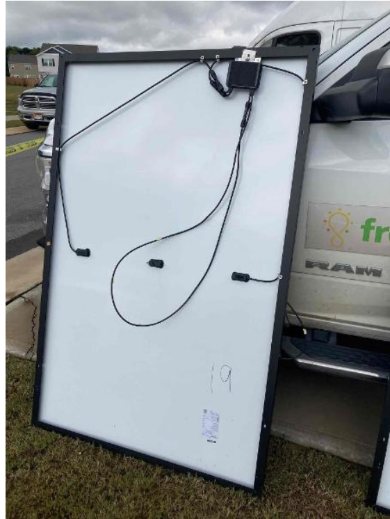
Rooftop Installation / Optimizer/ Micro Inverter Installed
