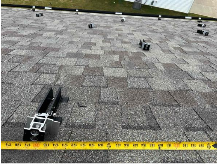
Rooftop Installation / Module Ready Photos
