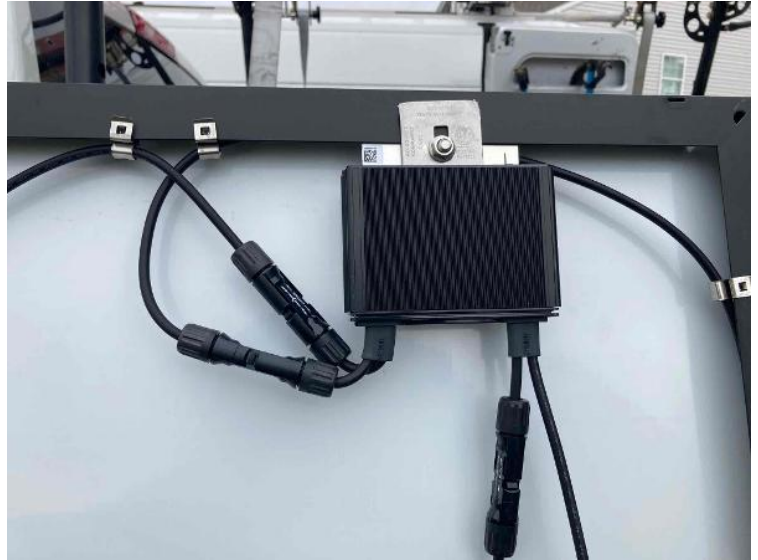
Rooftop Installation / Optimizer/ Micro Inverter Installed
