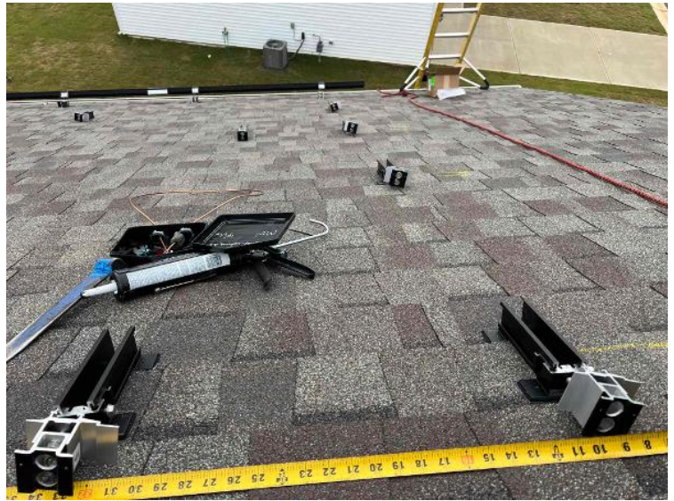
Rooftop Installation / Module Ready Photos
