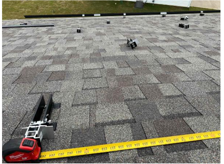
Rooftop Installation / Module Ready Photos
