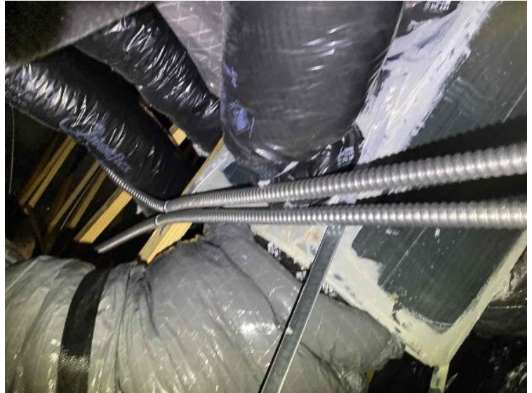
Rooftop Installation / Entire Attic Run
