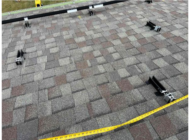
Rooftop Installation / Module Ready Photos
