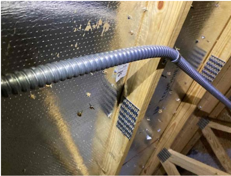
Rooftop Installation / Entire Attic Run
