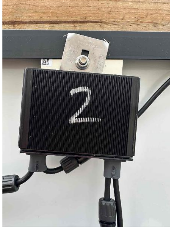
Rooftop Installation / Optimizer/ Micro Inverter Installed
