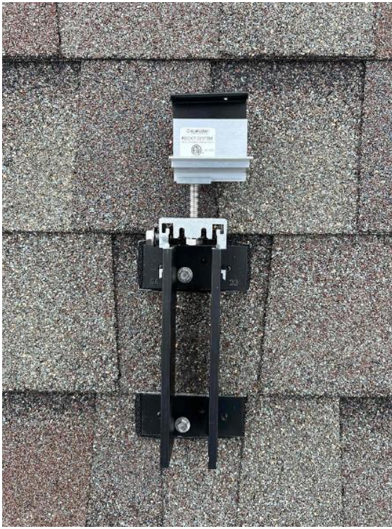
Rooftop Installation / Completed Roof Attachment
