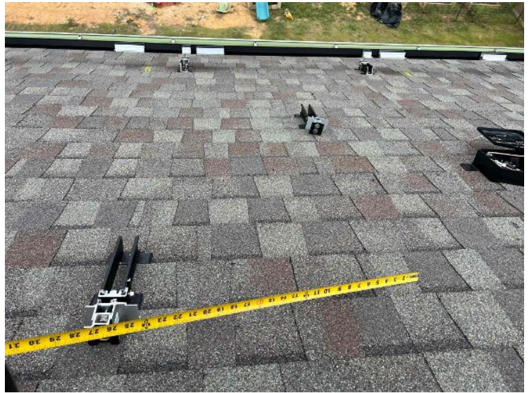
Rooftop Installation / Module Ready Photos
