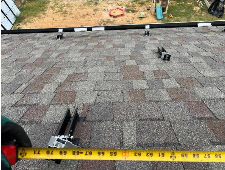
Rooftop Installation / Module Ready Photos
