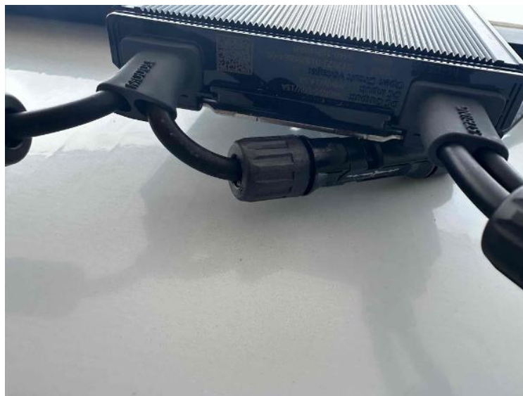
Rooftop Installation / Optimizer/ Micro Inverter Installed
