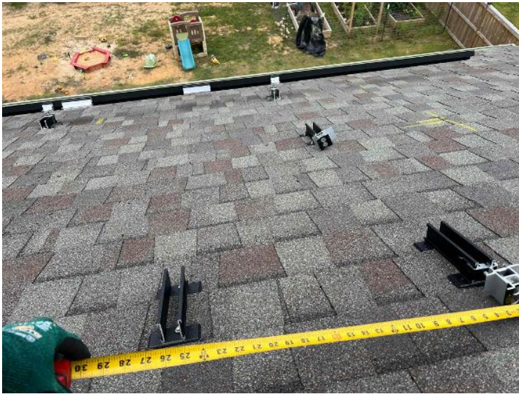
Rooftop Installation / Module Ready Photos
