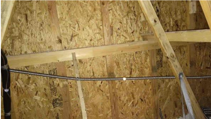
Rooftop Installation / Entire Attic Run
