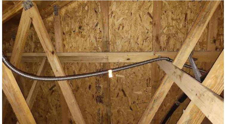
Rooftop Installation / Entire Attic Run
