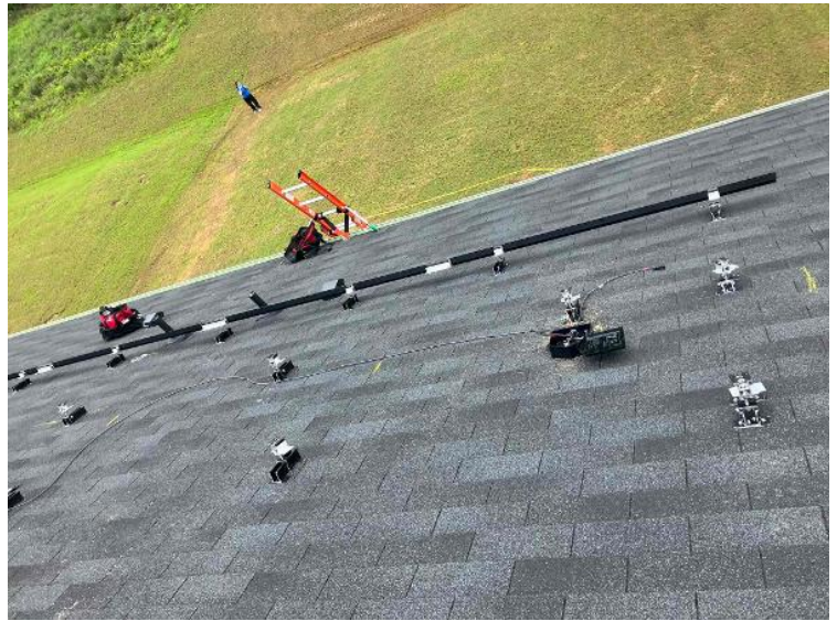
Rooftop Installation / Module Ready Photos
