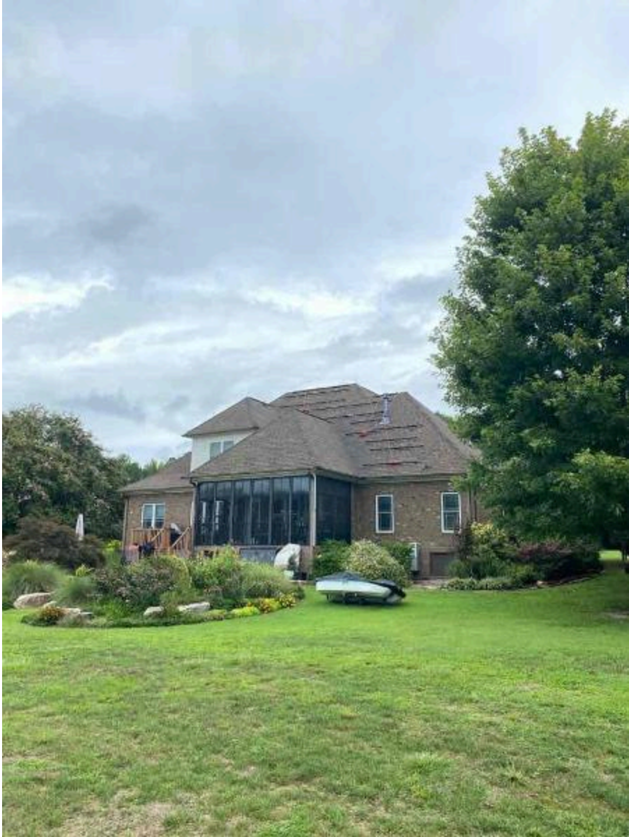
Photos for Inspection: 151 Fieldstone Dr, Holly Springs, NC 27540, USA
