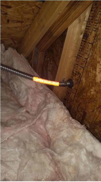
Rooftop Installation / Conduit Support Installed (Close-up Photos)
