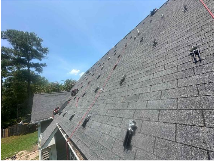
Rooftop Installation / Module Ready Photos
