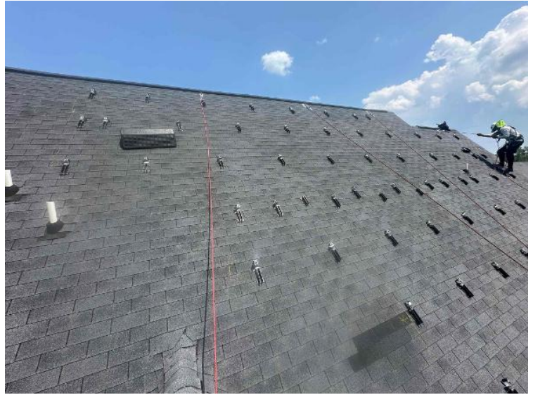
Rooftop Installation / Module Ready Photos
