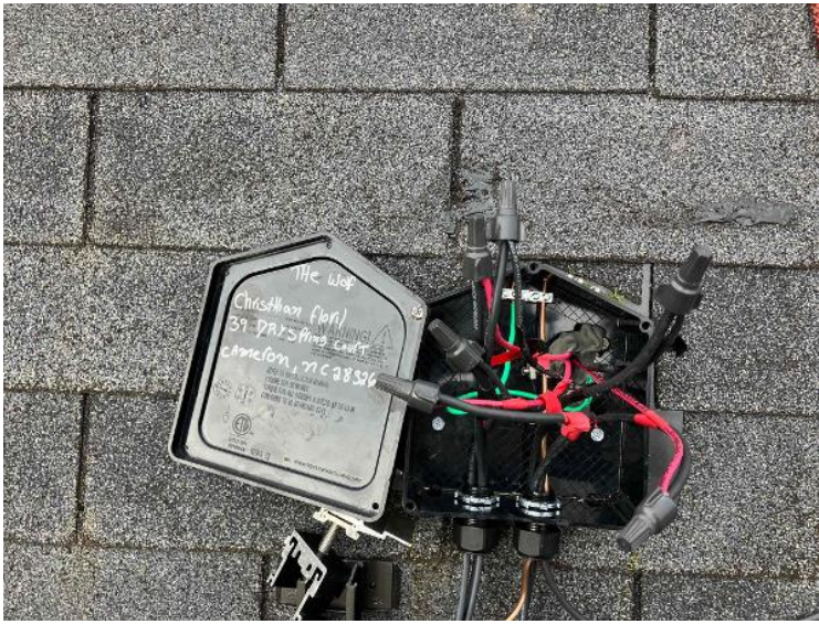
Rooftop Installation / J-Box Installed W/ Wiring Complete (All Components)
