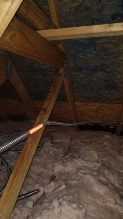
Rooftop Installation / Overall Conduit Run, Between Arrays, Attic Runs Included, Down To BOS
