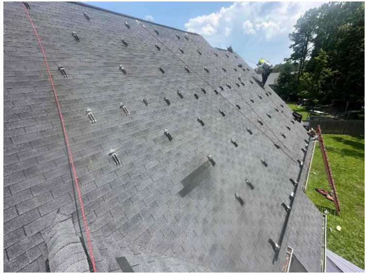
Rooftop Installation / Module Ready Photos
