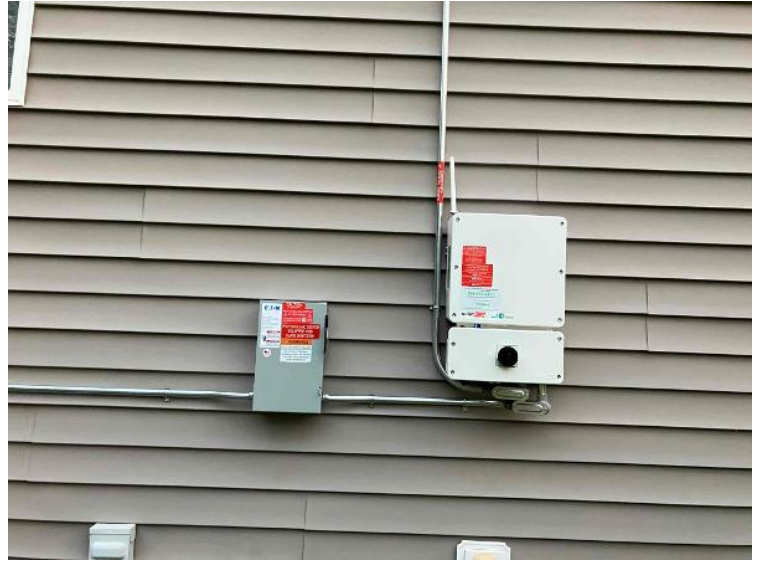
Rooftop Installation / Conduit Support Installed (Close-up Photos)
