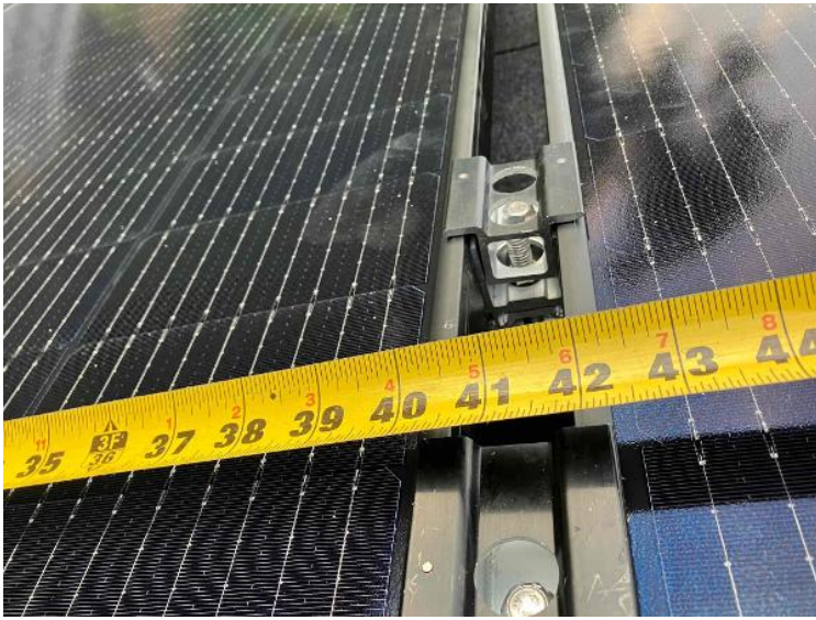
Rooftop Installation / Module Gapping: Tape Measure showing 3/8" - 1" Gap
