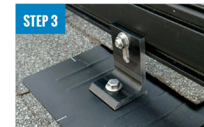
ATTACH L-FOOT TO RAIL
