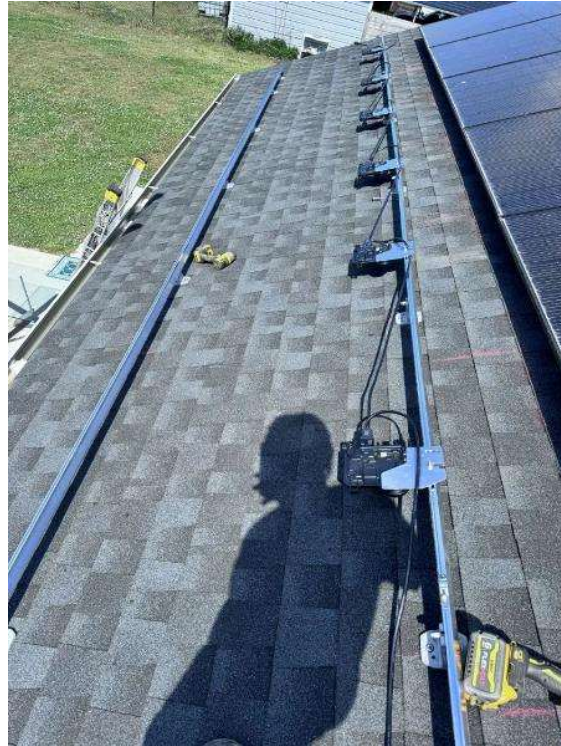
Roof Photos (All Photos with a * by them are required for panel pay bonus) / Upclose Photos of Splices
