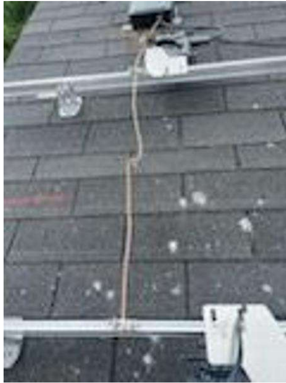
Roof Photos (All Photos with a * by them are required for panel pay bonus) / Uplclose photos of Rack Grounding
