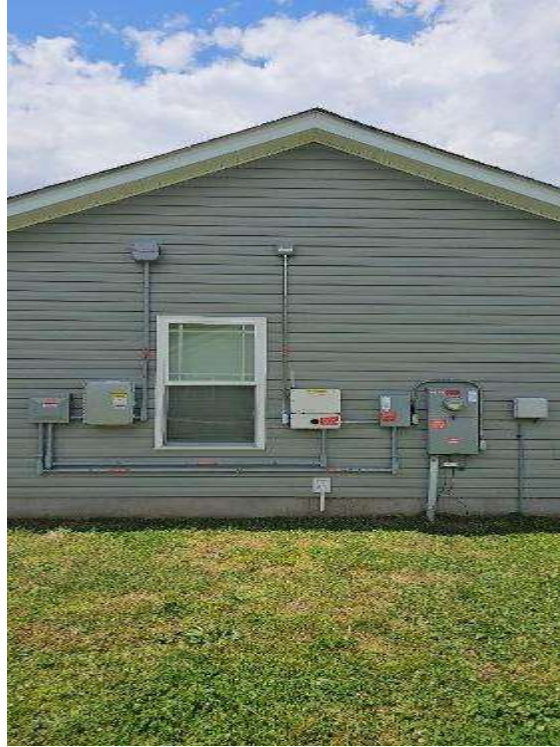
Electrical Photos (All Photos with a * by them are required for panel pay bonus) / Dry wall need to be repaired? Show photo. If not, show that it doesnt
