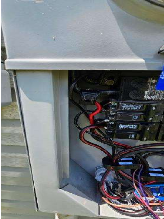
Electrical Photos (All Photos with a * by them are required for panel pay bonus) / Line Or Load Side Tap
