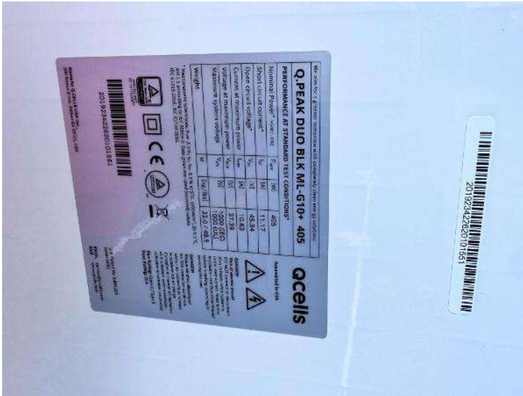
Roof Photos (All Photos with a * by them are required for panel pay bonus) / Module Label, Brand and Size. (The Module label on the back of the panel)
