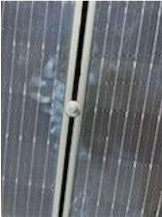
Roof Photos (All Photos with a * by them are required for panel pay bonus) / Uplclose photos of Mids and Ends
