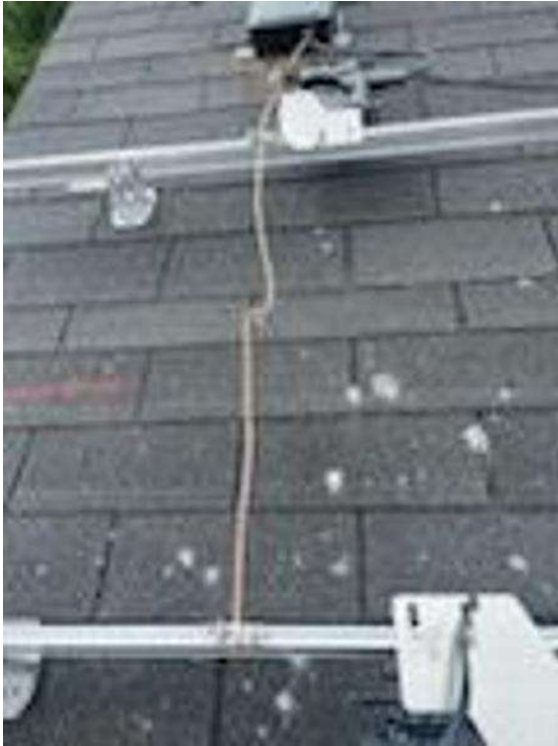
Roof Photos (All Photos with a * by them are required for panel pay bonus) / Every 2' of Grounding before panels
