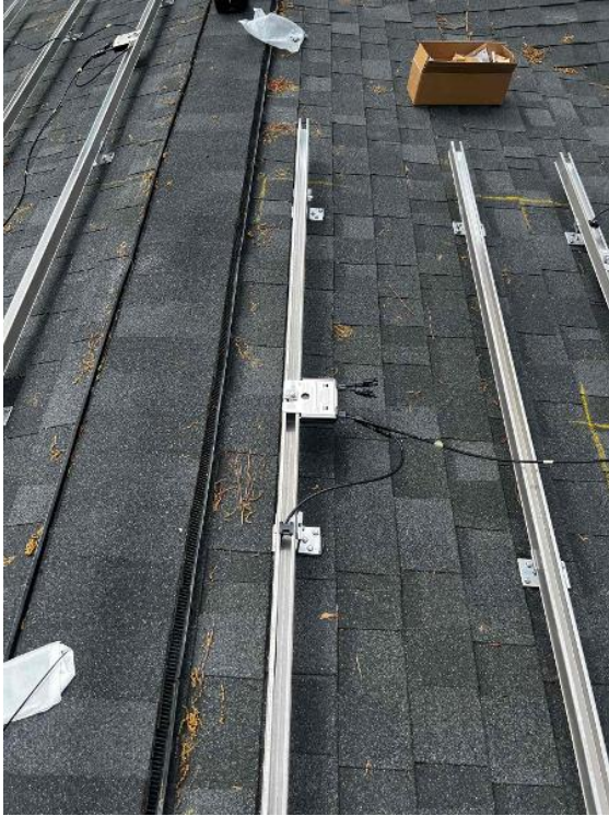
Array / Grounding: 1) Take an up close photo of the rail bonding lug along with panned out photos of the entire ground wire.
