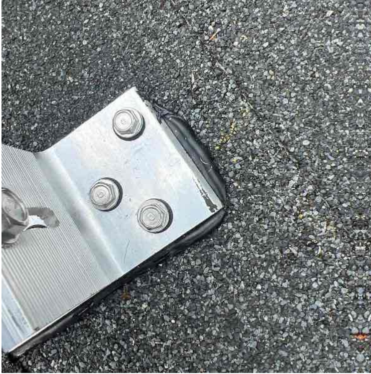
Roof Leak Prevention / Photo of at least 1 flashing with sealant applied in the correct U-shape
