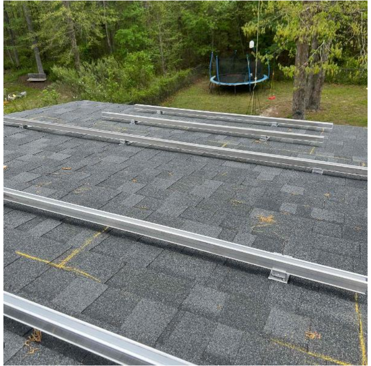
Array / Roof Attachment and Racking Layout - showing COMPLETE layouts, staggered attachments, span measurement. (2 pics per array min) If this is a tile roof get some clear photos of the tile condition before laying panels.
