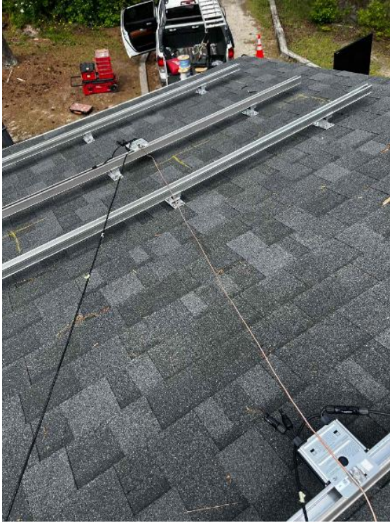
Array / Grounding: 1) Take an up close photo of the rail bonding lug along with panned out photos of the entire ground wire.
