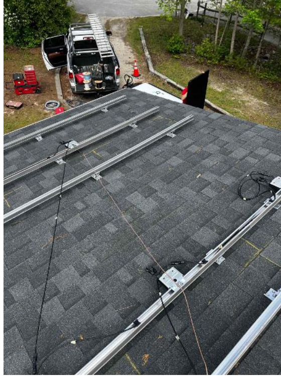
Array / Grounding: 1) Take an up close photo of the rail bonding lug along with panned out photos of the entire ground wire.
