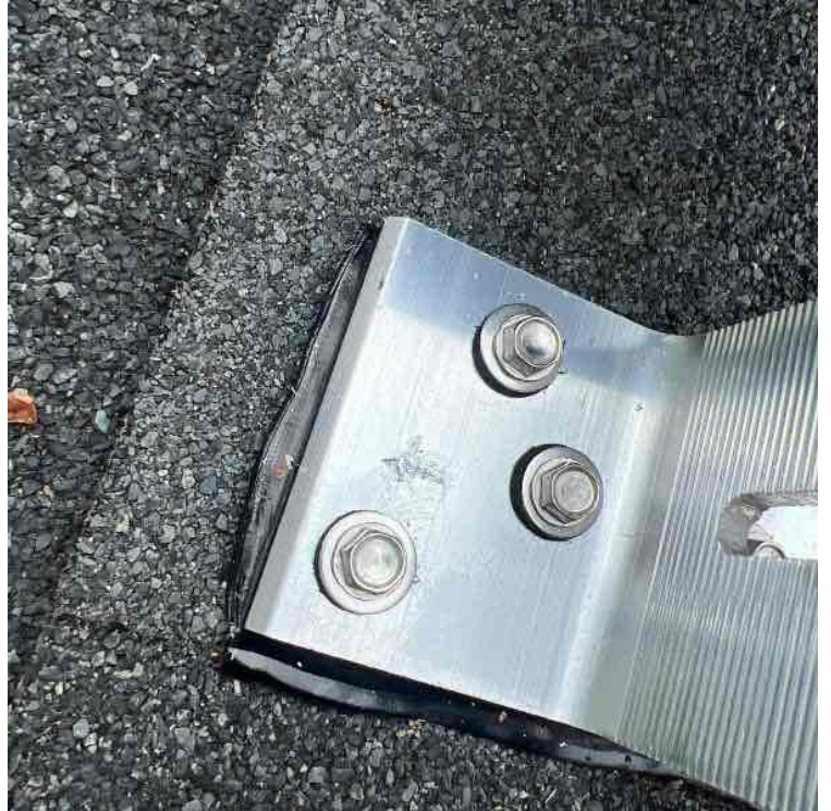
Roof Leak Prevention / Photo of at least 1 flashing with sealant applied in the correct U-shape
