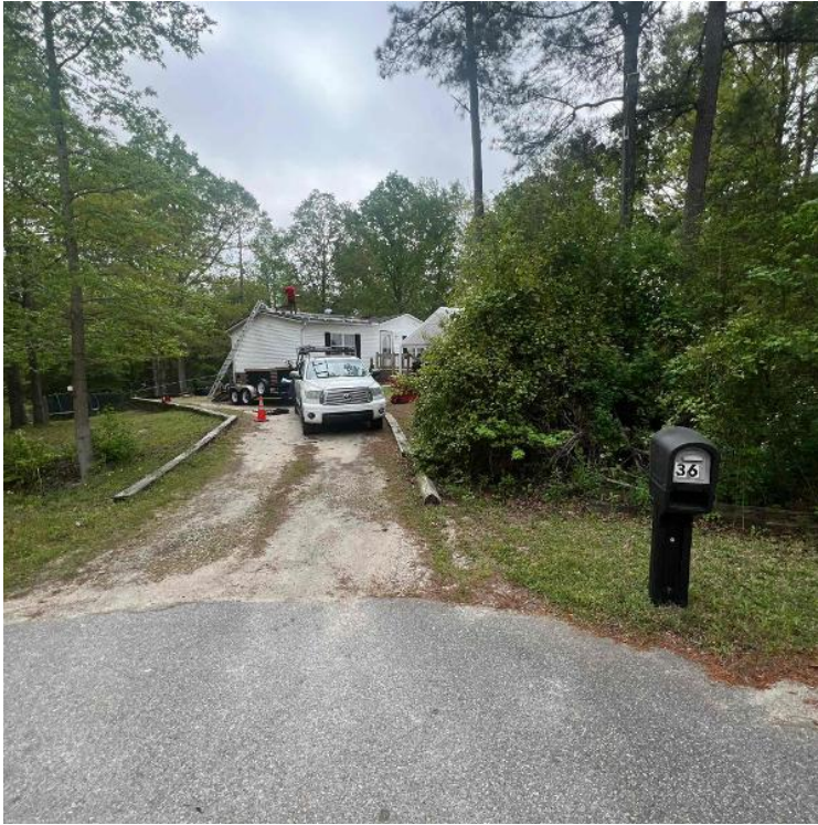
Job Setup / Location - Show front of home
