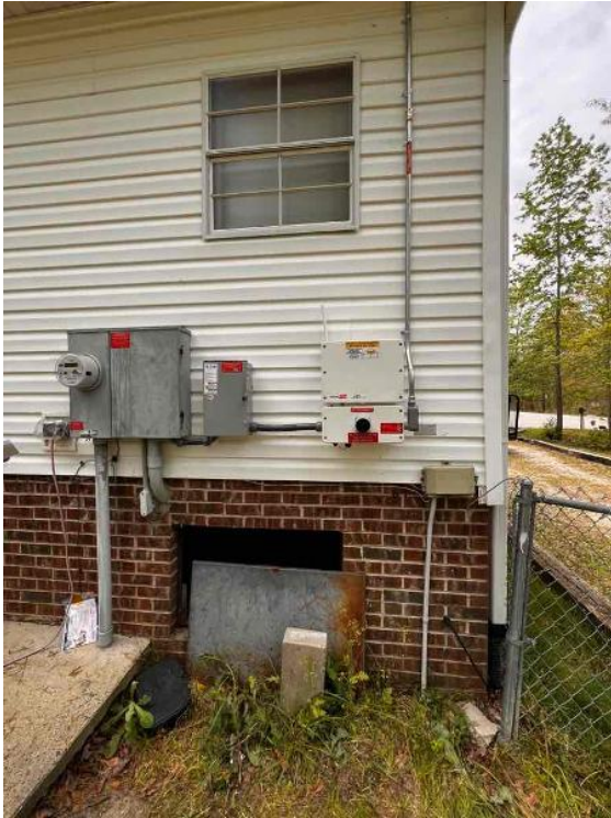
Electrical / Photo of location of plans left on site
