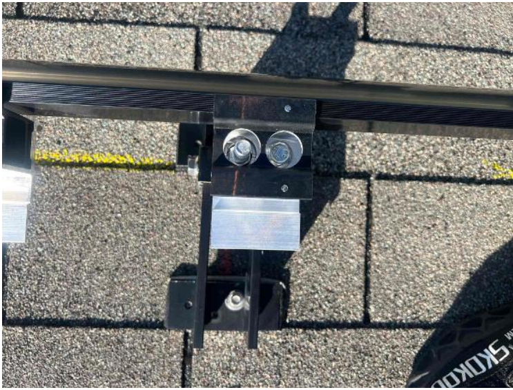
Rooftop Installation / Completed Roof Attachment
