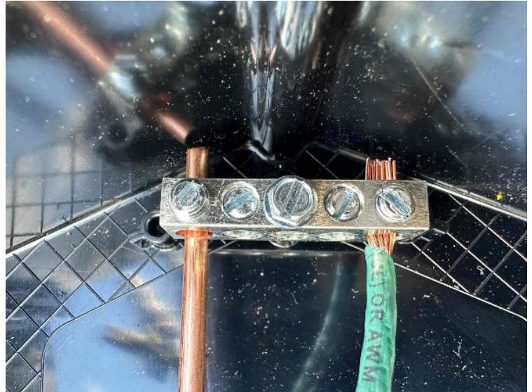
Rooftop Installation / Array Bonding/Grounding
