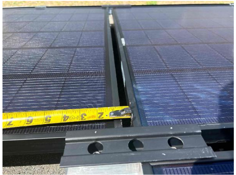
Rooftop Installation / Module Gapping: Tape Measure showing 3/8" - 1" Gap
