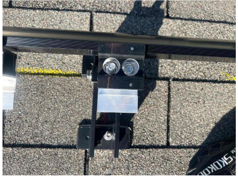
Rooftop Installation / Module Ready Photos
