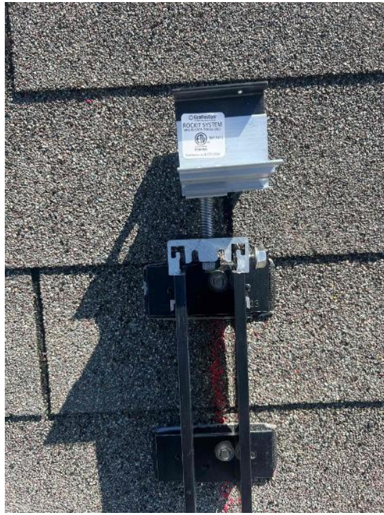
Rooftop Installation / Completed Roof Attachment
