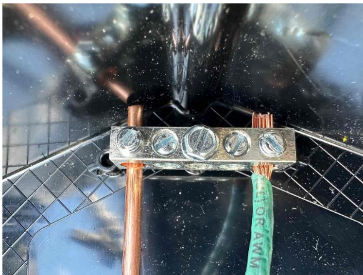
Rooftop Installation / J-Box Installed W/ Wiring Complete (All Components)
