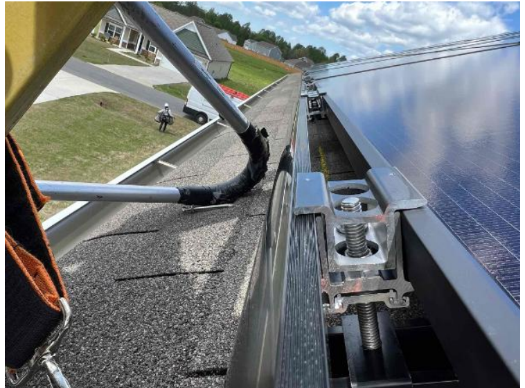
Rooftop Installation / Close Up of Skirt Splice + Skirt Roof Attachment Complete
