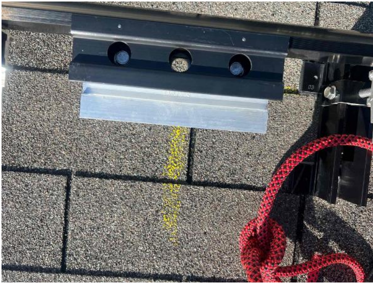
Rooftop Installation / Module Ready Photos
