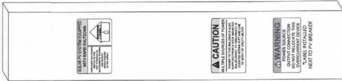
MAIN SERVICE PANEL
