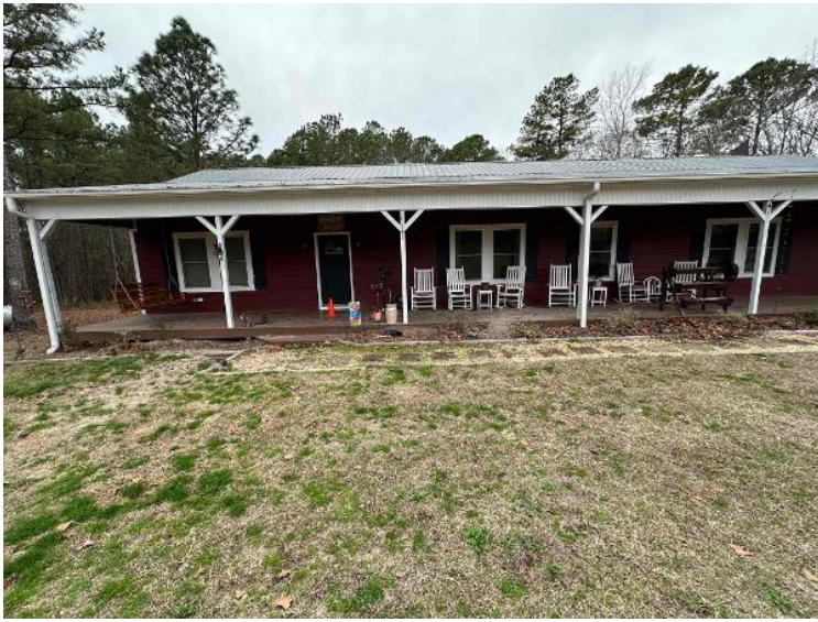
Job Check In / Picture of Front of the House
