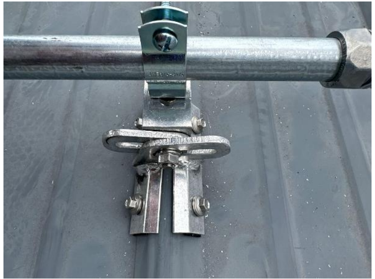
Rooftop Installation / Conduit Support Installed (Close-up Photos)
