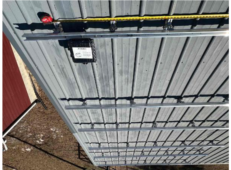
Rooftop Installation / Module Ready Photos
