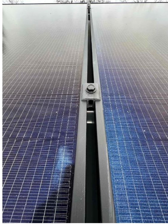
Rooftop Installation / Mid Clamps Installed (side view)
