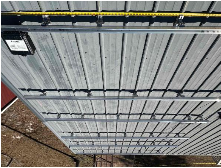
Rooftop Installation / Module Ready Photos
