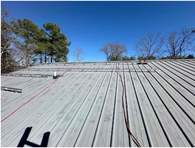
Rooftop Installation / Module Ready Photos
