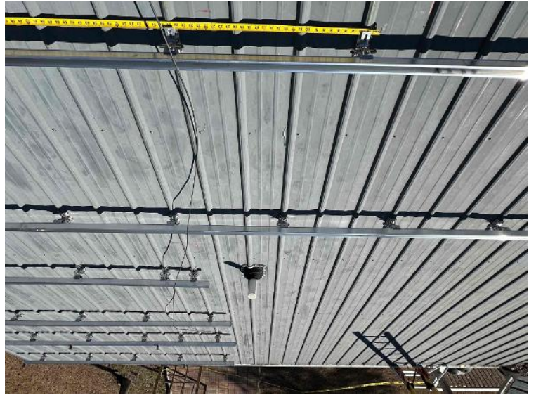
Rooftop Installation / Module Ready Photos
