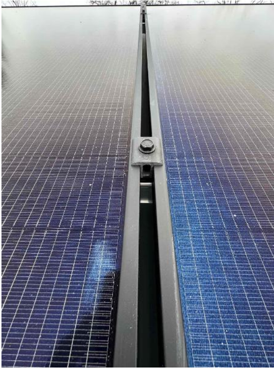
Rooftop Installation / Module Gapping: Tape Measure showing 3/8" - 1" Gap
