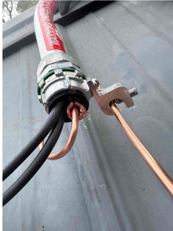
Rooftop Installation / Array Bonding/Grounding
