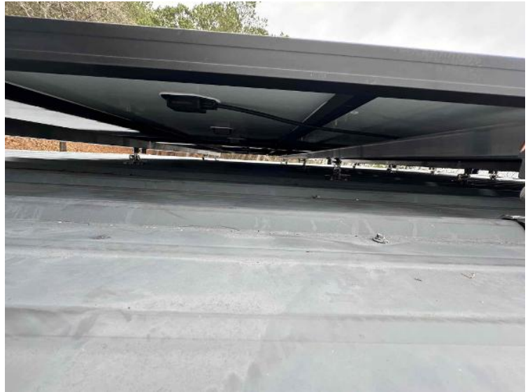
Rooftop Installation / Wire management Under the Array (1 photo per row of modules per array)
