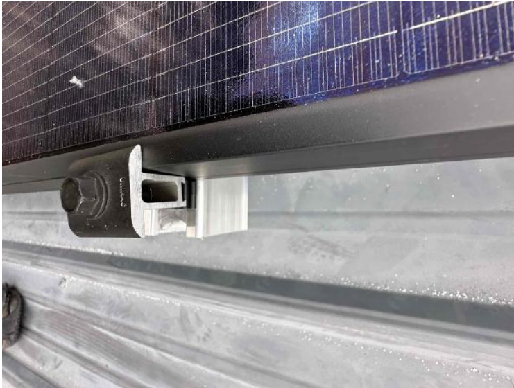
Rooftop Installation / End Clamp Engaged To Module
