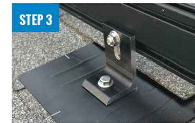
ATTACH L-FOOT TO RAIL
