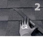
Locate, choose, and mark centers of rafters to be Carefully lift composition roof shingle with roofing Insert flashing between 1st and 2nd course. Slide mounted. Select the courses of shingles where bar, just above placement of mount. Remove up so top edge of flashing is at least ¾" higher nails as required and backfill holes with aproved than the butt-edge of the 3rd course and lower sealant. See "Proper Flashing Placement" on next flashing edge is above the butt-edge of 1st course
