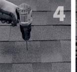
If attaching with lag bolt use a 📆 "bit (Lag). Use a Clean off any sawdust, and fill hole with sealant Place L-foot onto elevated flute and rotate L-foot to 1/8" bit (ST) for attaching with the structural screw. compatible with roofing materials. Drill pilot hole into roof and rafter, taking care to drill square to the roof. Do not use mount as a drill guide. Drill a 2" deep hole into rafter.
