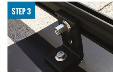
ATTACH L-FOOT TO RAIL
