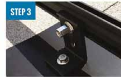
ATTACH L-FOOT TO RAIL
