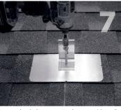
Prepare lag bolt or structural screw with sealing You are now ready for the rack of your choice. washer. Using a ½-inch socket on an impact gun, drive prepared lag bolt through L-foot until L-foot can no longer easily rotate. DO NOT over-torque. NOTE: Structural screw can be driven with T-30 hex head bit.
