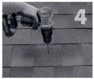
If attaching with lag bolt use a 📆 "bit (Lag). Use a Clean off any sawdust, and fill hole with sealant Place L-foot onto elevated flute and rotate L-foot to 1/8" bit (ST) for attaching with the structural screw. compatible with roofing materials. Drill pilot hole into roof and rafter, taking care to drill square to the roof. Do not use mount as a drill guide. Drill a 2" deep hole into rafter.
