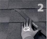
Locate, choose, and mark centers of rafters to be Carefully lift composition roof shingle with roofing Insert flashing between 1st and 2nd course. Slide mounted. Select the courses of shingles where bar, just above placement of mount. Remove up so top edge of flashing is at least ¾" higher nails as required and backfill holes with aproved than the butt-edge of the 3rd course and lower sealant. See "Proper Flashing Placement" on next flashing edge is above the butt-edge of 1st course
