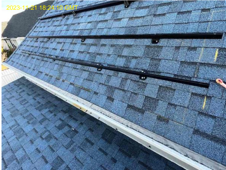
Roof/Array Information / Roof Array / Picture of feet installed on roof
