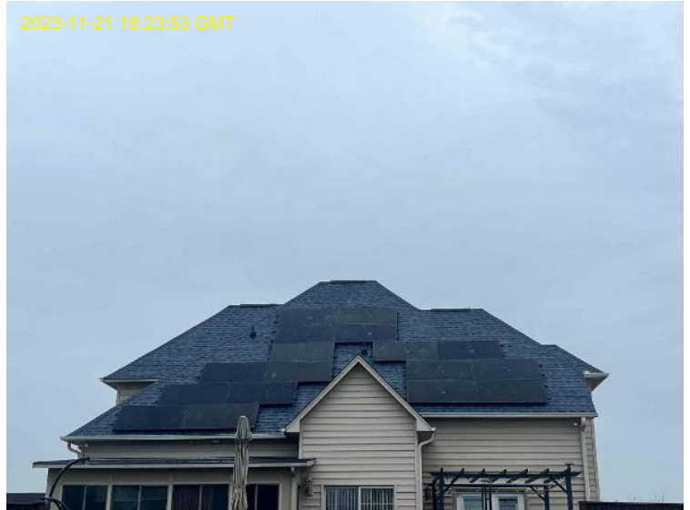
Roof/Array Information / Roof Array / Photo of completed array
