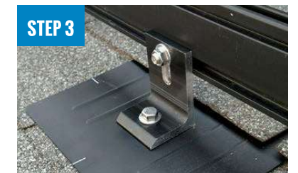
STEP 3 ATTACH L-FOOT TO RAIL
