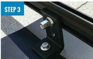
ATTACH L-FOOT TO RAIL
