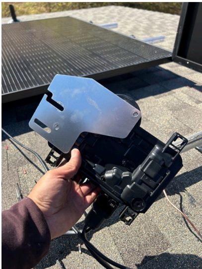
Detailed picture of micro inverter W/ reference point in background of model info
