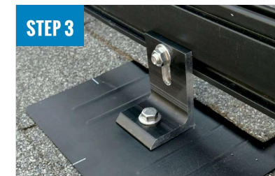
ATTACH L-FOOT TO RAIL
