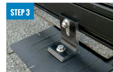
ATTACH L-FOOT TO RAIL
