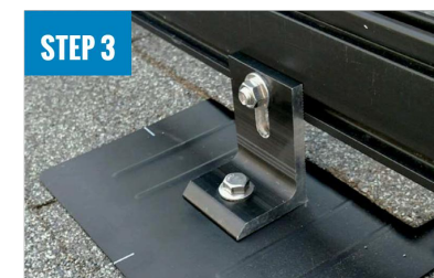
ATTACH L-FOOT TO RAIL
