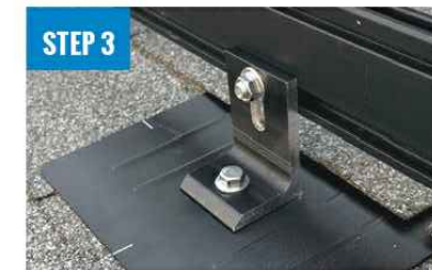
ATTACH L-FOOT TO RAIL
