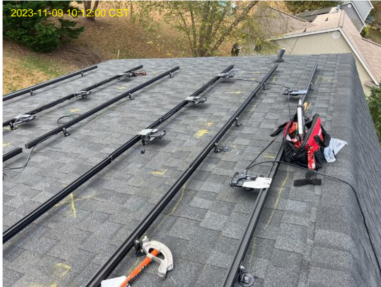
Rail / U Series Array Racking - MIs Installed
