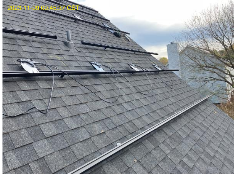
Rail / U Series Array Racking - MIs Installed
