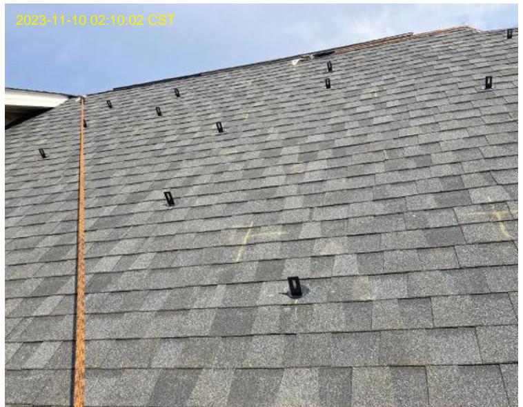
Roof Attachments / Wide Shot of Roof Attachment
