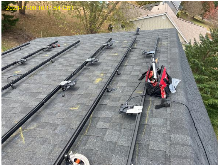
Rail / U Series Array Racking - MIs Installed
