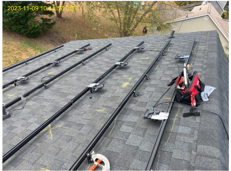
Rail / U Series Array Racking - MIs Installed
