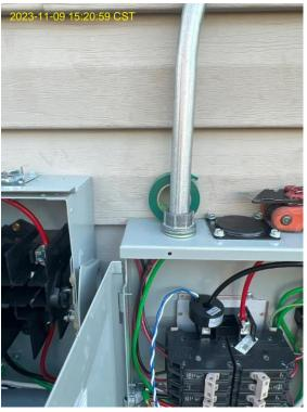
$\operatorname{EMT}/\operatorname{Close}$  Up of Tightened Couplers, Connectors, & Nipples.
