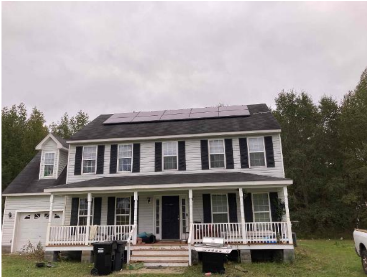
Project Completion Photos / Complete Array Photos (all modules can be counted in each array)
