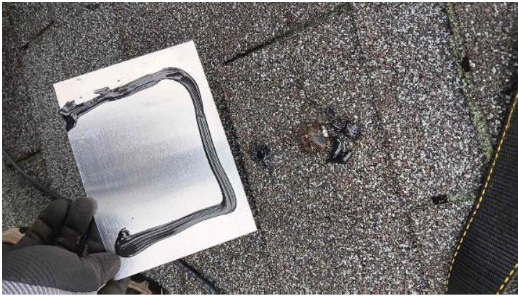
Waterproofing All Penetrations / PPE Anchor Penetrations Sealed
