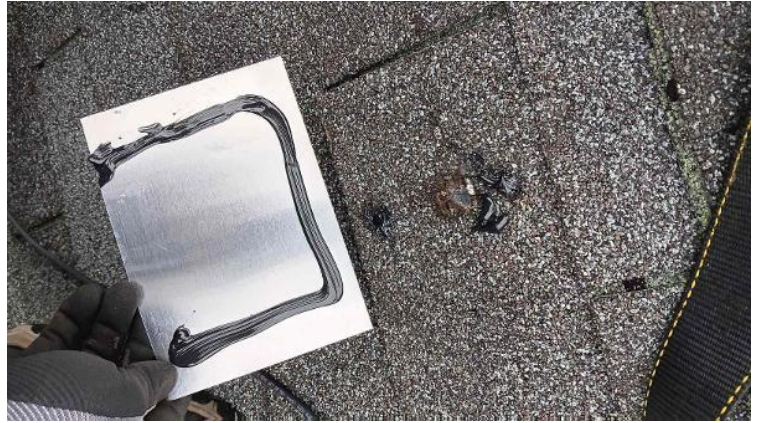
Waterproofing All Penetrations / U-Shape of Sealant Applied to the Flashing
