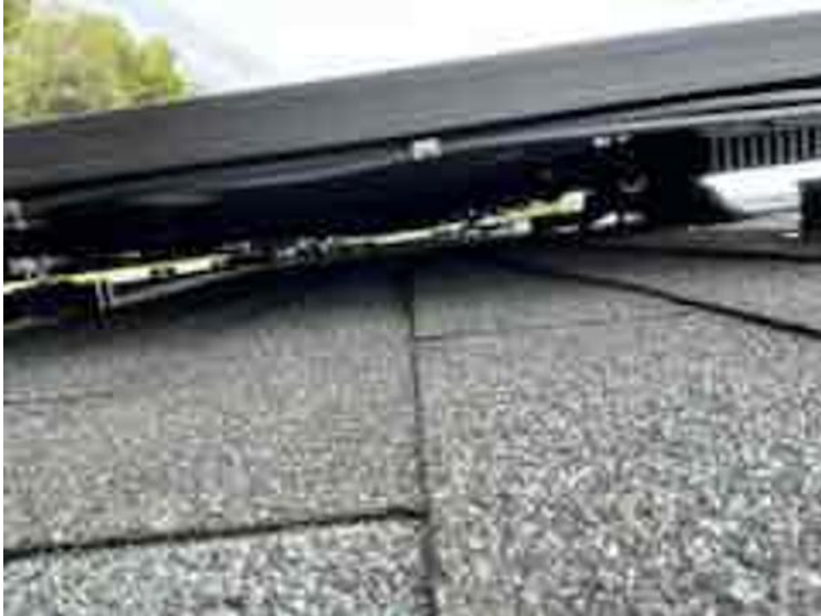
Module Installation / Wire management Under the Array (1 photo per row of modules per array)
