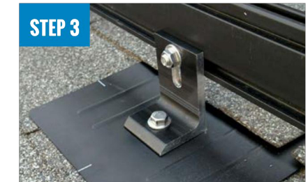
ATTACH L-FOOT TO RAIL
