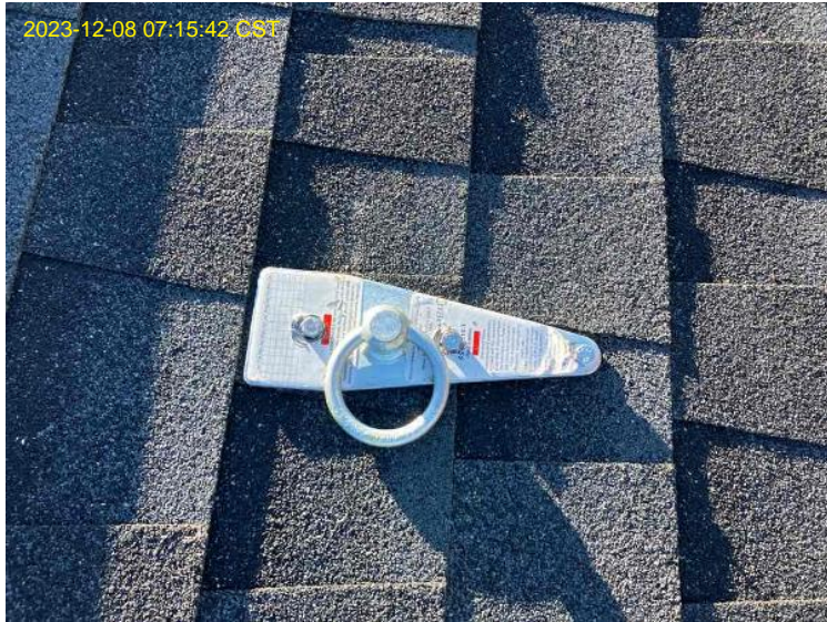
Anchor / Fall Protection Anchor (Fastened into the rafters w/ all 3 lag screws used)
