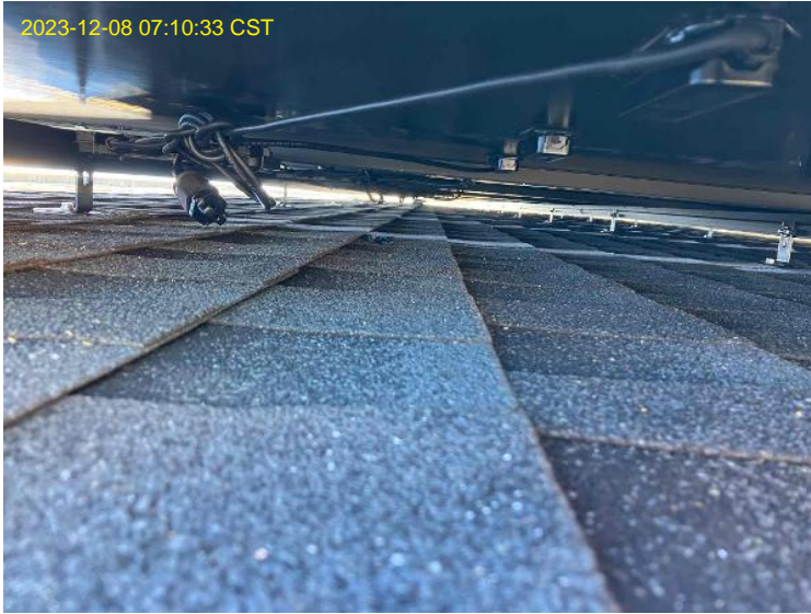
Modules / Wire Management - Under Array (Must be taken from ROOF)
