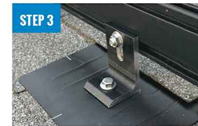
ATTACH L-FOOT TO RAIL
