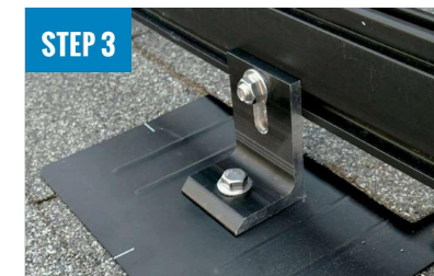
ATTACH L-FOOT TO RAIL
