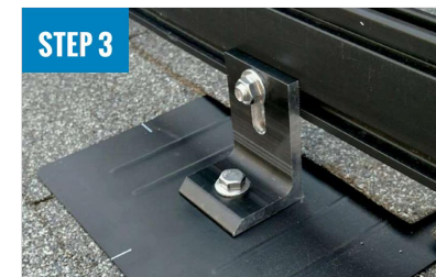
ATTACH L-FOOT TO RAIL
