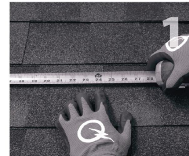
1 Locate, choose, and mark centers of rafters to be mounted. Select the courses of shingles where mounts will be placed.
