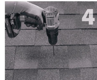
4 If attaching with lag bolt use a 1/4" (Lag). Use a 1/8" bit (ST) for attaching with the structural screw. Drill pilot hole into roof and rafter, taking care to drill square to the roof. Do not use mount as a drill guide. Drill a 2" deep hole into rafter.
