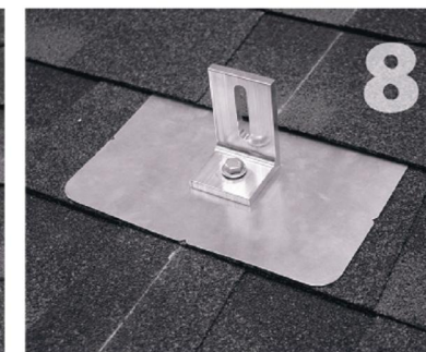
8 You are now ready for the rack of your choice. Follow all the directions of the rack manufacturer as well as the module manufacturer. NOTE: Make sure top of L-Foot makes solid contact with racking.
