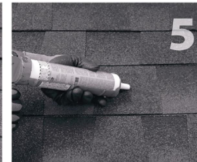
5 Clean off any sawdust, and fill hole with sealant compatible with roofing materials.
