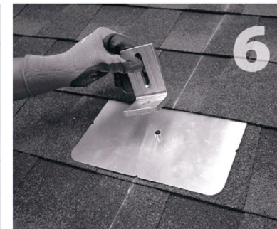
6 Place L-foot onto elevated flange and rotate L-foot to desired orientation.
