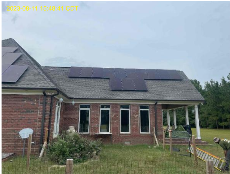
Roof/Array Work / Photo: Overall Array (s)
