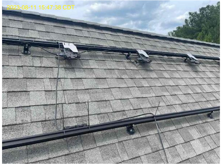
Roof/Array Work / Photo: Flashing/Roof Mount wide shot (racking)
